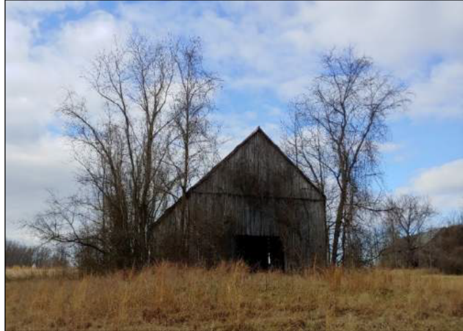
Figure 4: One of the tobacco barns located on the Forney Farm. The second barn can be seen in the background to the right.
