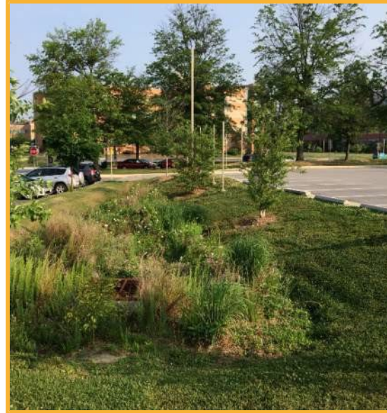
Example micro-scale ESD / water quality facility
