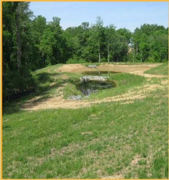
Example stormwater quantity management facility
