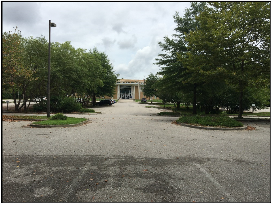
Figure 2. Looking east towards the library from the parking lot
