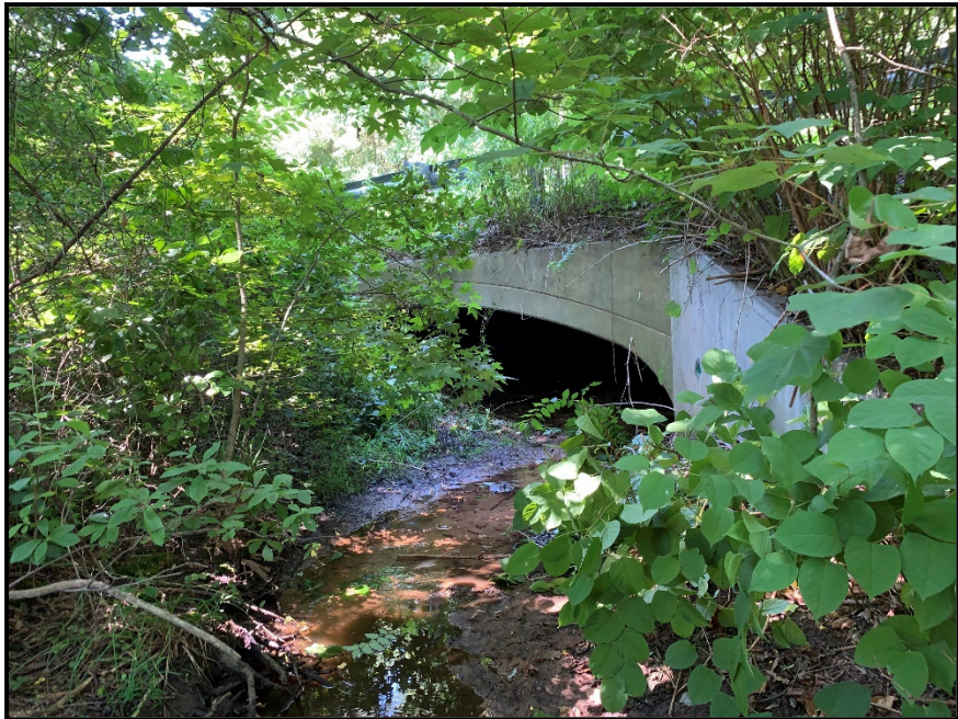
Figure 8. Existing culvert under Winmeyer Avenue
