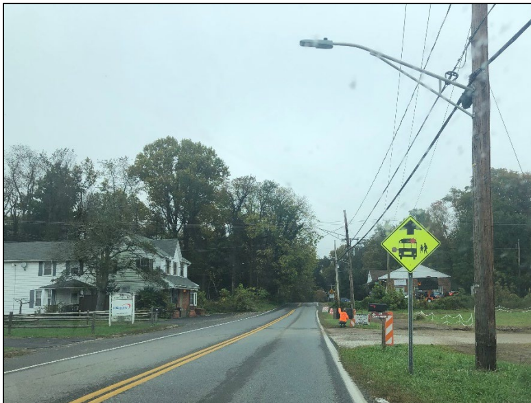
Gambrills Road, facing north toward future South Shore Trail crossing
