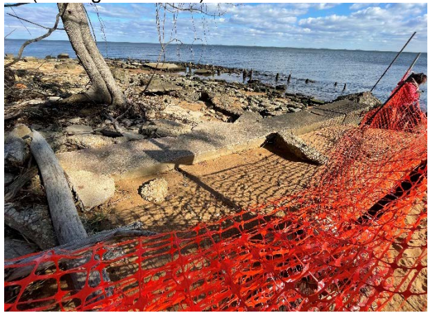
Photo 3 – Concrete Wall at North End
