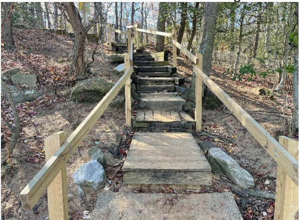
Photo 2 - Stairs leading to Dog Beach Area
