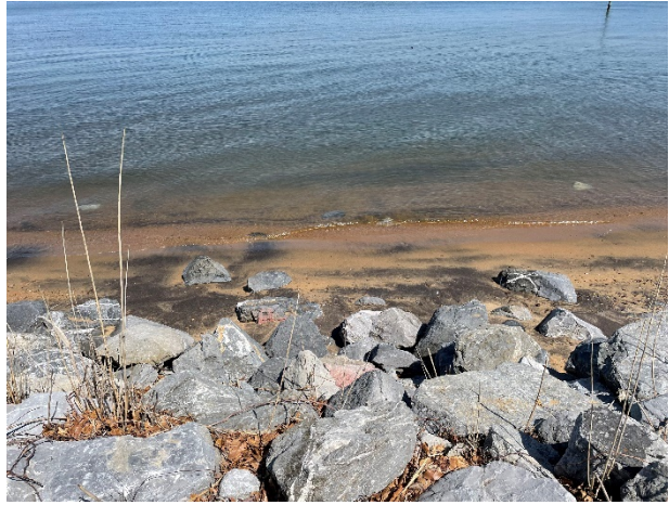
Photo 16 – Stones Scattered Seaward of Structure
