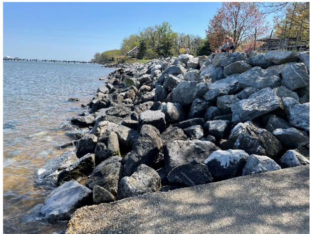
Photo 20 – Larger Revetment at Northern End (looking South)
