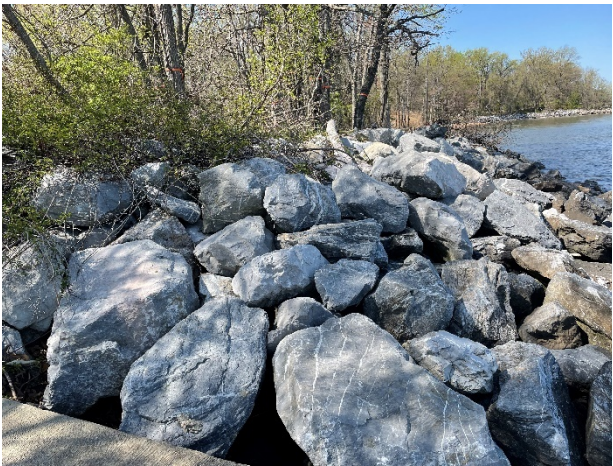
Photo 19 – Larger Revetment at Northern End (looking North)
