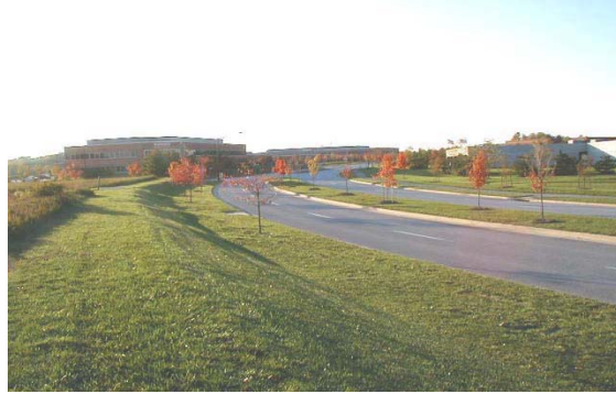
Wide roadways lined with trees
