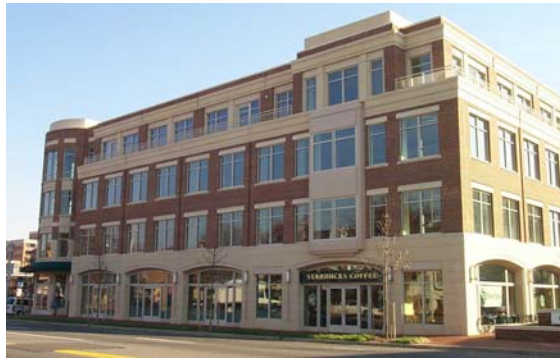
Office buildings set to the sidewalk
