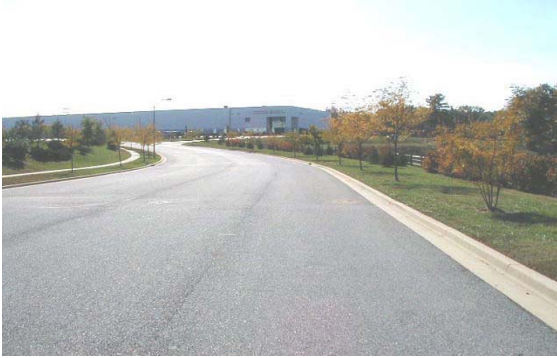
Large warehouse buildings sited to minimize visual impact on the surroundings
