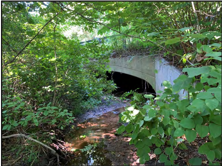
Figure 8. Existing culvert under Winmeyer Avenue
