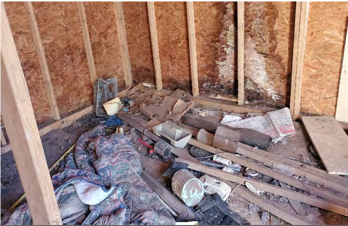
Interior of wooden structure
