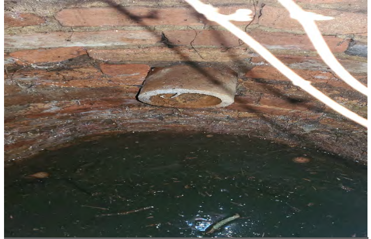
Terracotta piping and liquid in cistern/pit
