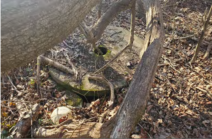
Cistern/Pit – Northeast portion of the Site
