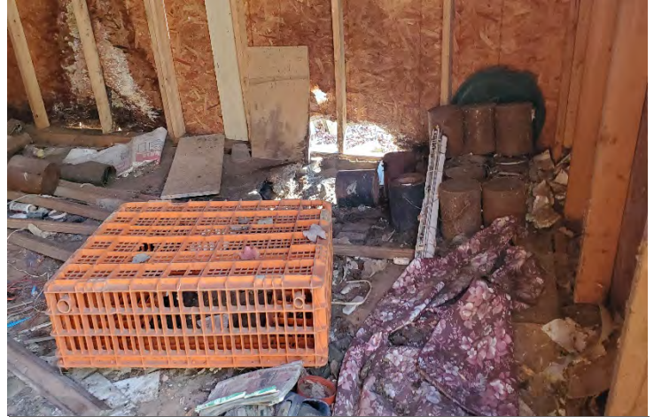
Interior of wooden structure
