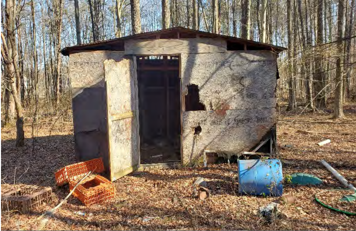
Wooden structure and miscellaneous trash
