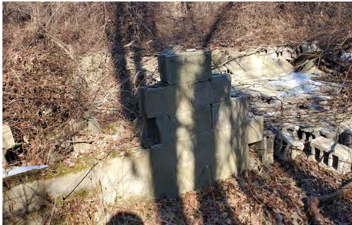
Remains of a former structure – Northeast portion of the Site
