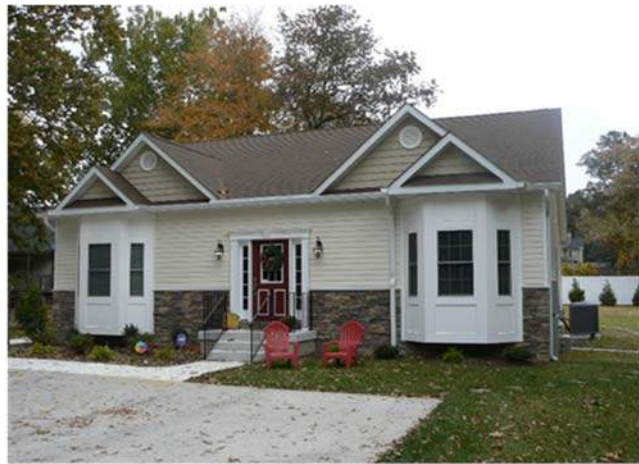
Human Services Renovations
