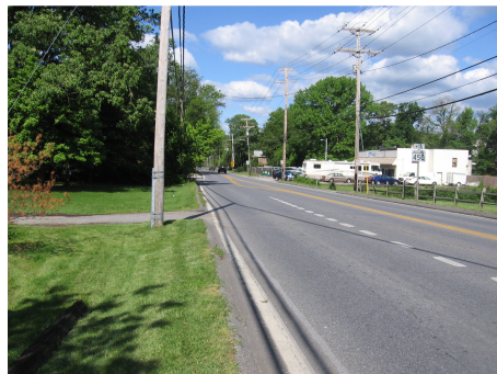
Lack of Sidewalk on MD 450 West
