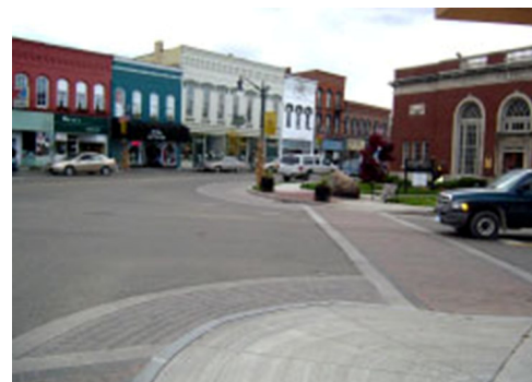
Colored, textured treatments were used on driving surfaces to alert motorists as they enter a pedestrian setting.
