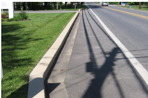
New curb cuts and shoulders
