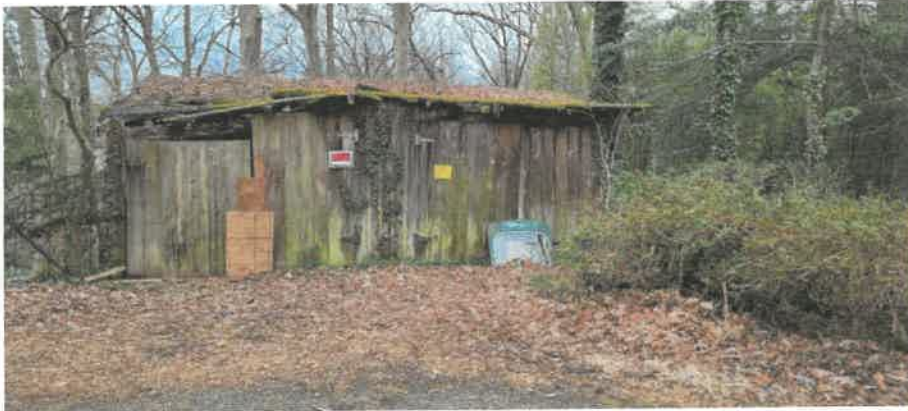
Existing Shed front
