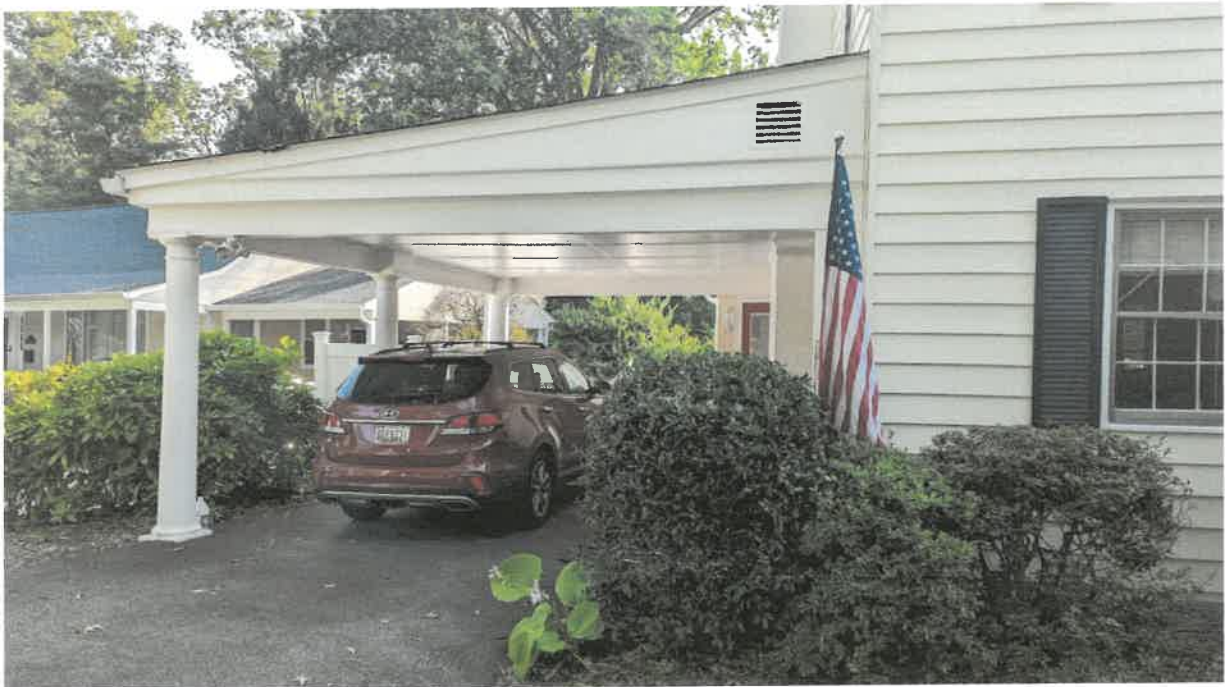
Figure 1: Carport showing existing columns and framing
