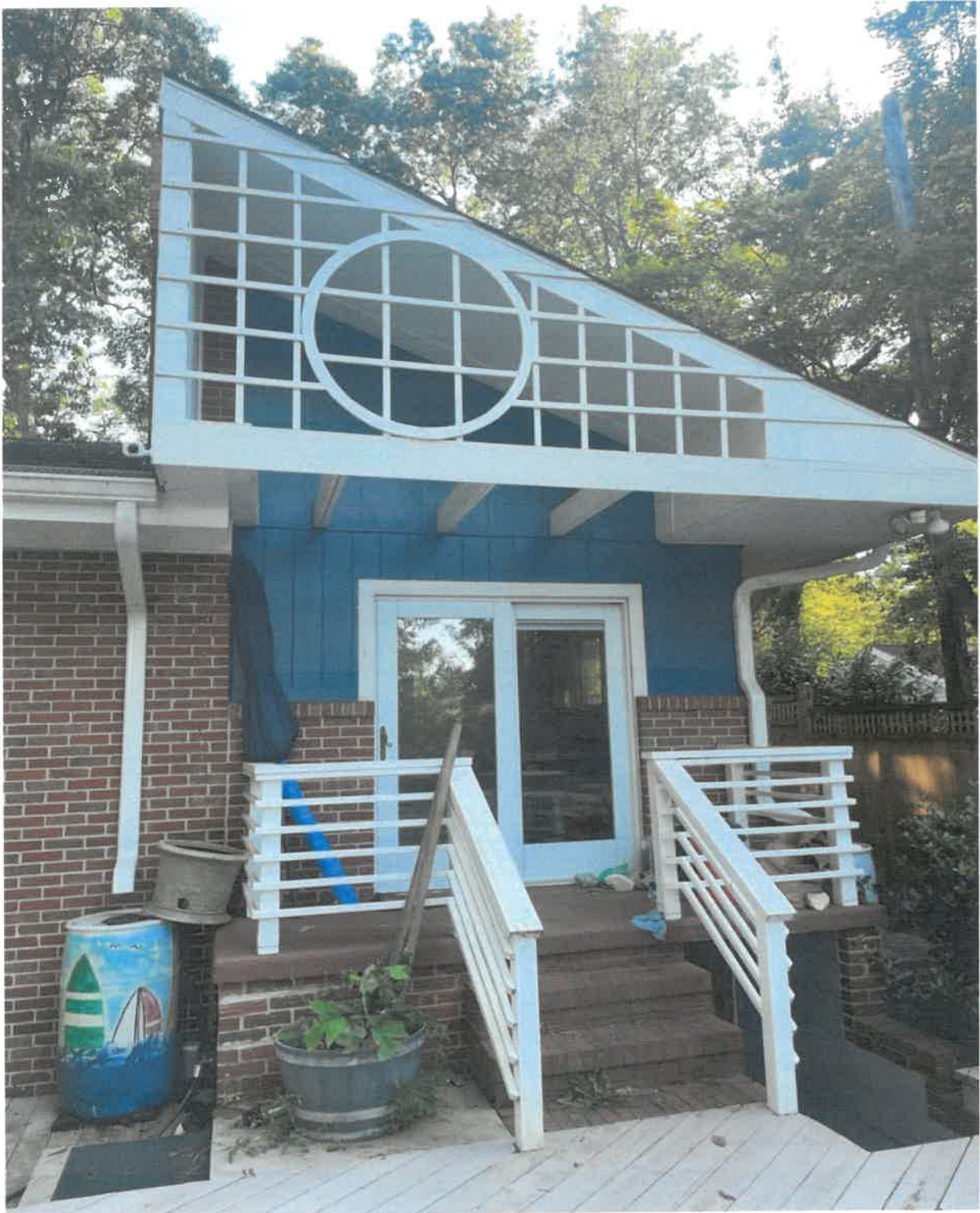
Photo of rear of existing home porch to remain.
