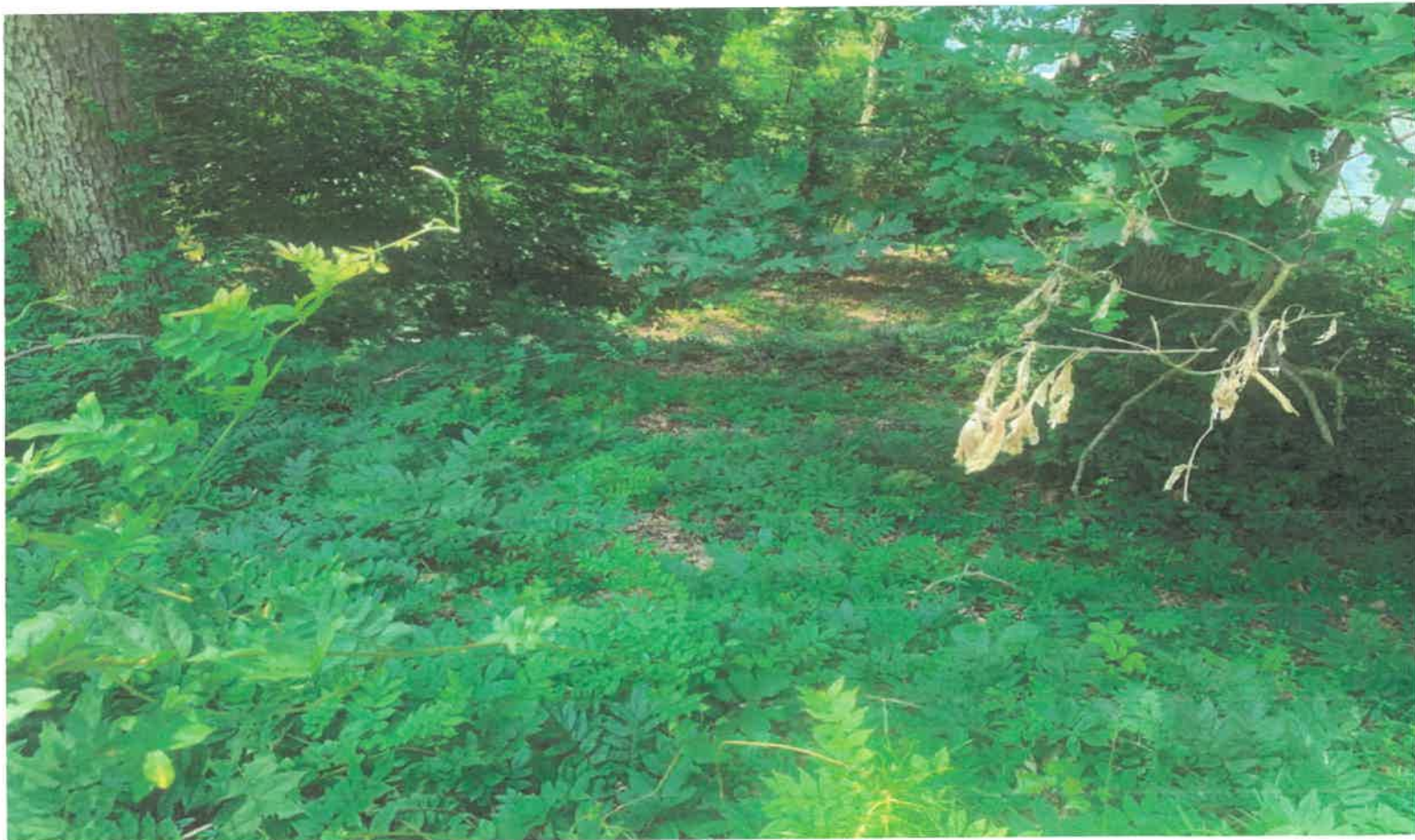
Photo #2 Looking South Down Existing Slope, No Erosion Present. Area Is Vegetatively Stabilized
