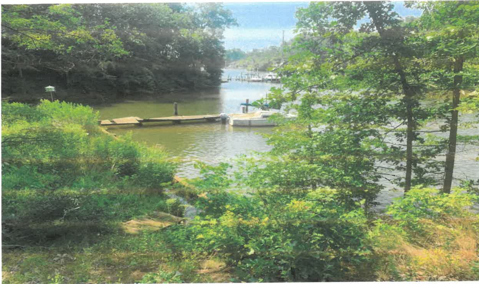
Photo #23 Looking Southwest Towards Gingerville Creek, No Erosion Present & Area Stabilized
