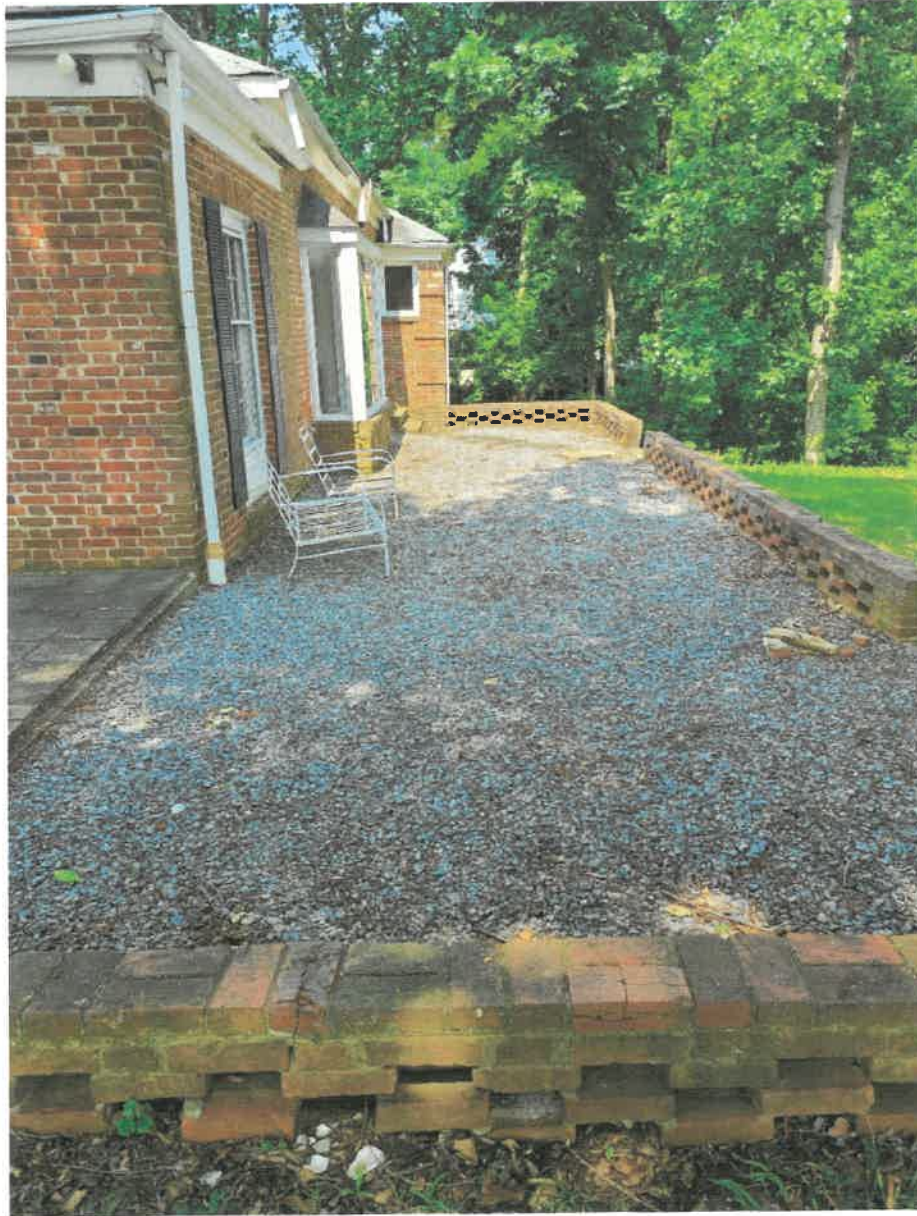
LOOKING NORTHEAST AT EXISTING NORTH SIDE BRICK WALL AND GRAVEL PATIO
