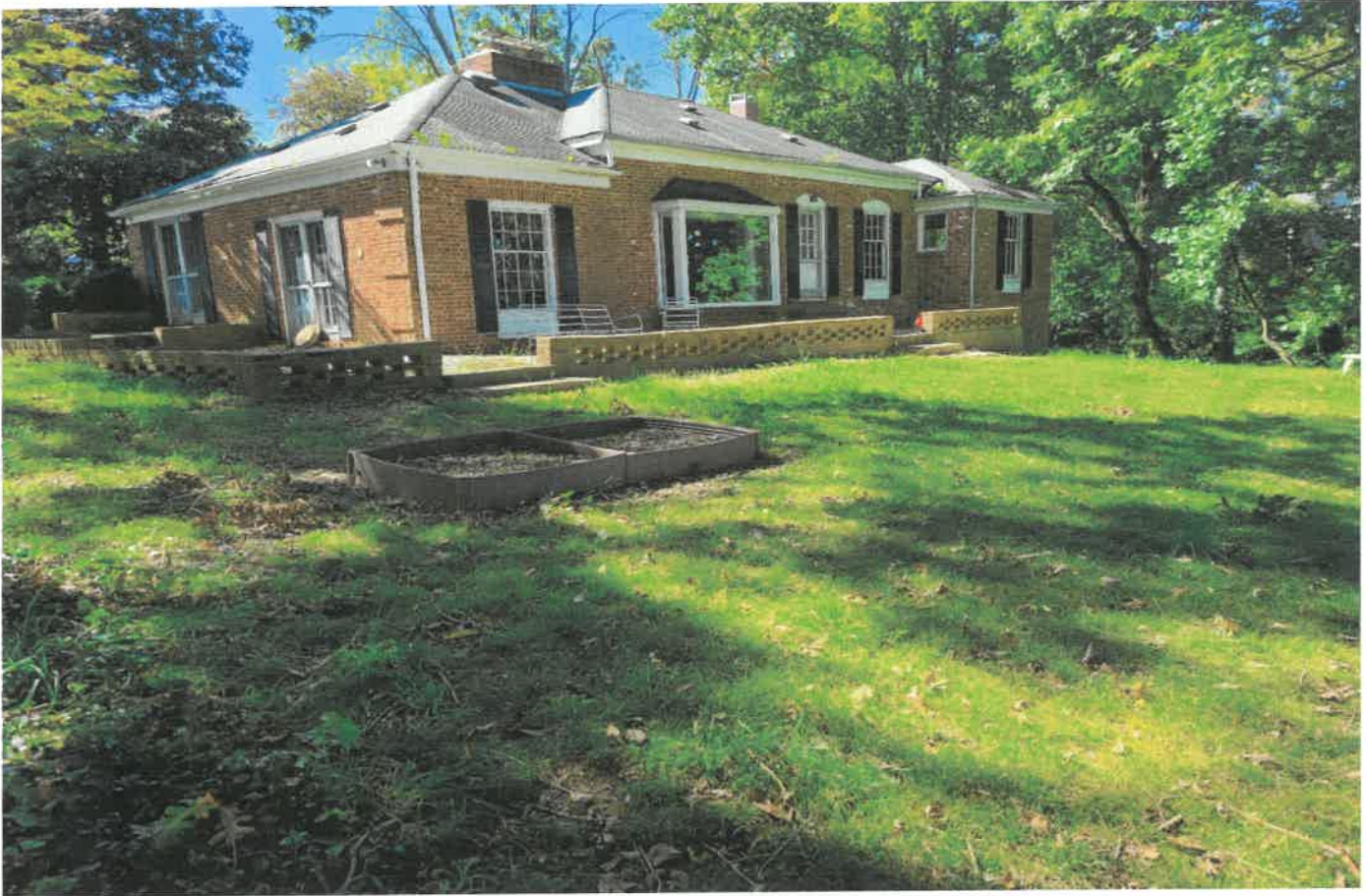
LOOKING SOUTHWEST AT NORTHEAST SIDE OF THE EXISTING HOUSE & PATIOS
