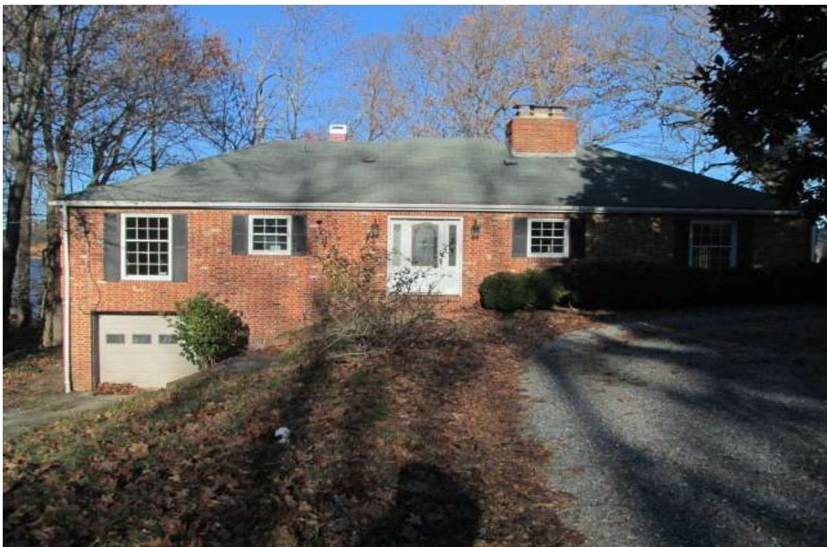
LOOKING NORTH AT SOUTH SIDE OF THE EXISTING HOUSE & DRIVEWAY
