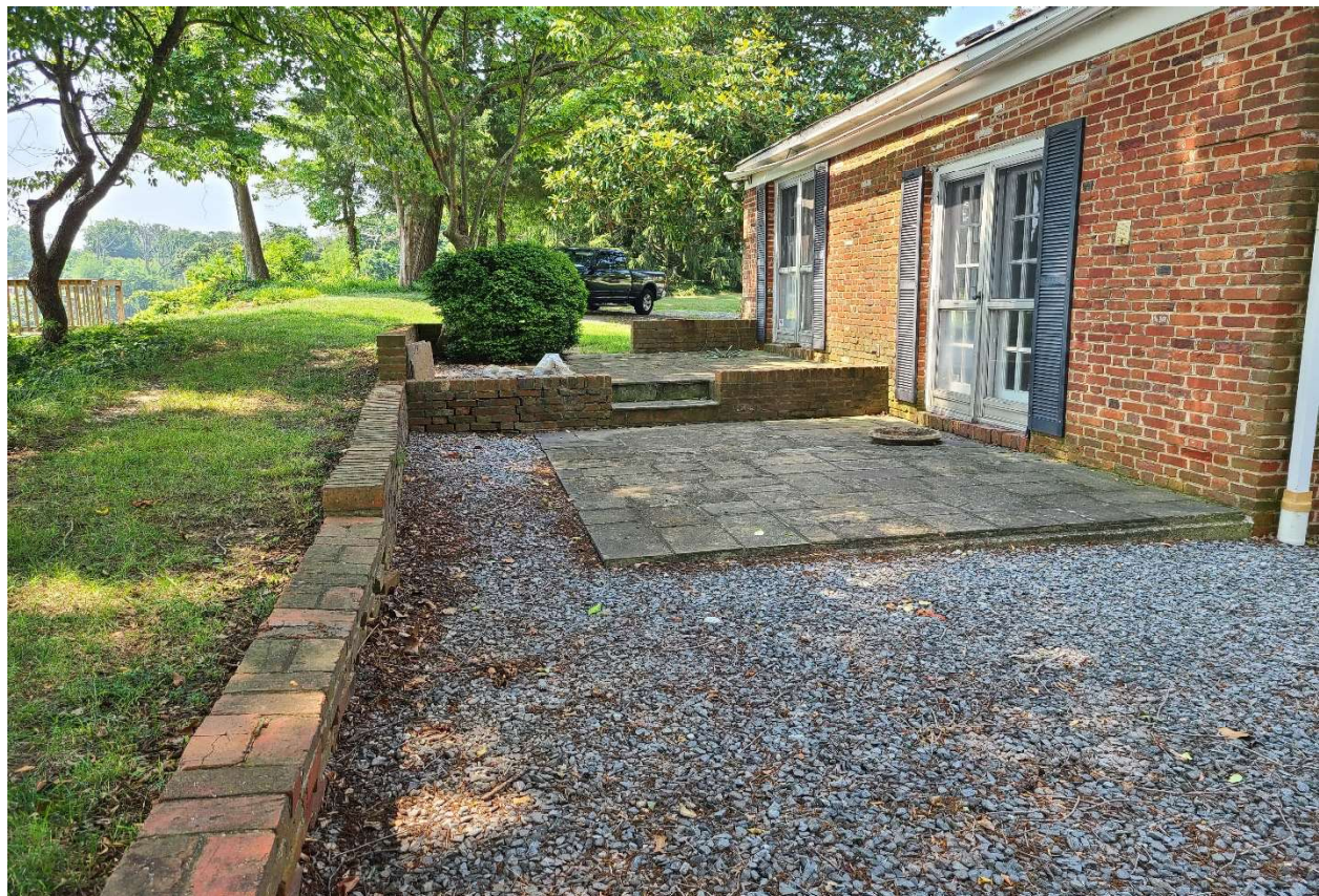
EXISTING EAST SIDE BRICK WALL AND GRAVEL SLATE PATIO
