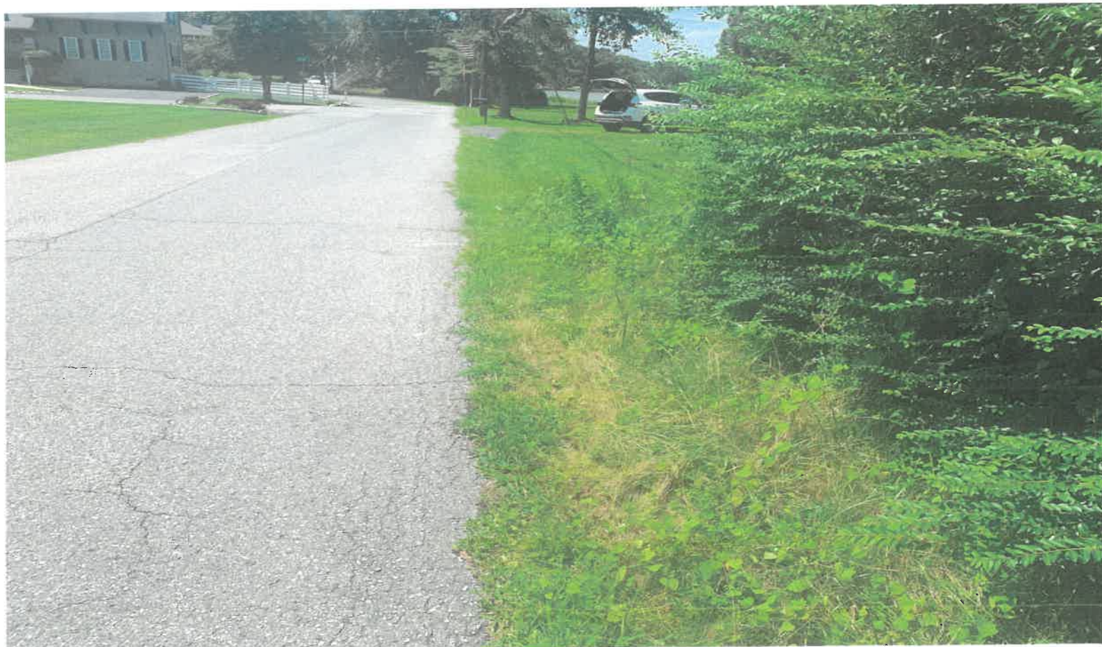
Existing Drainage Swale Running Along Side Southern Property Line
