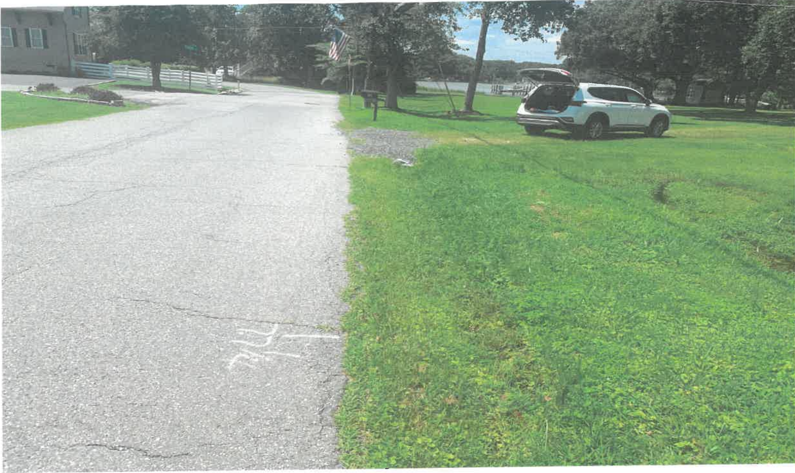
Existing Swale Approaching Subject Properties Existing Drive
