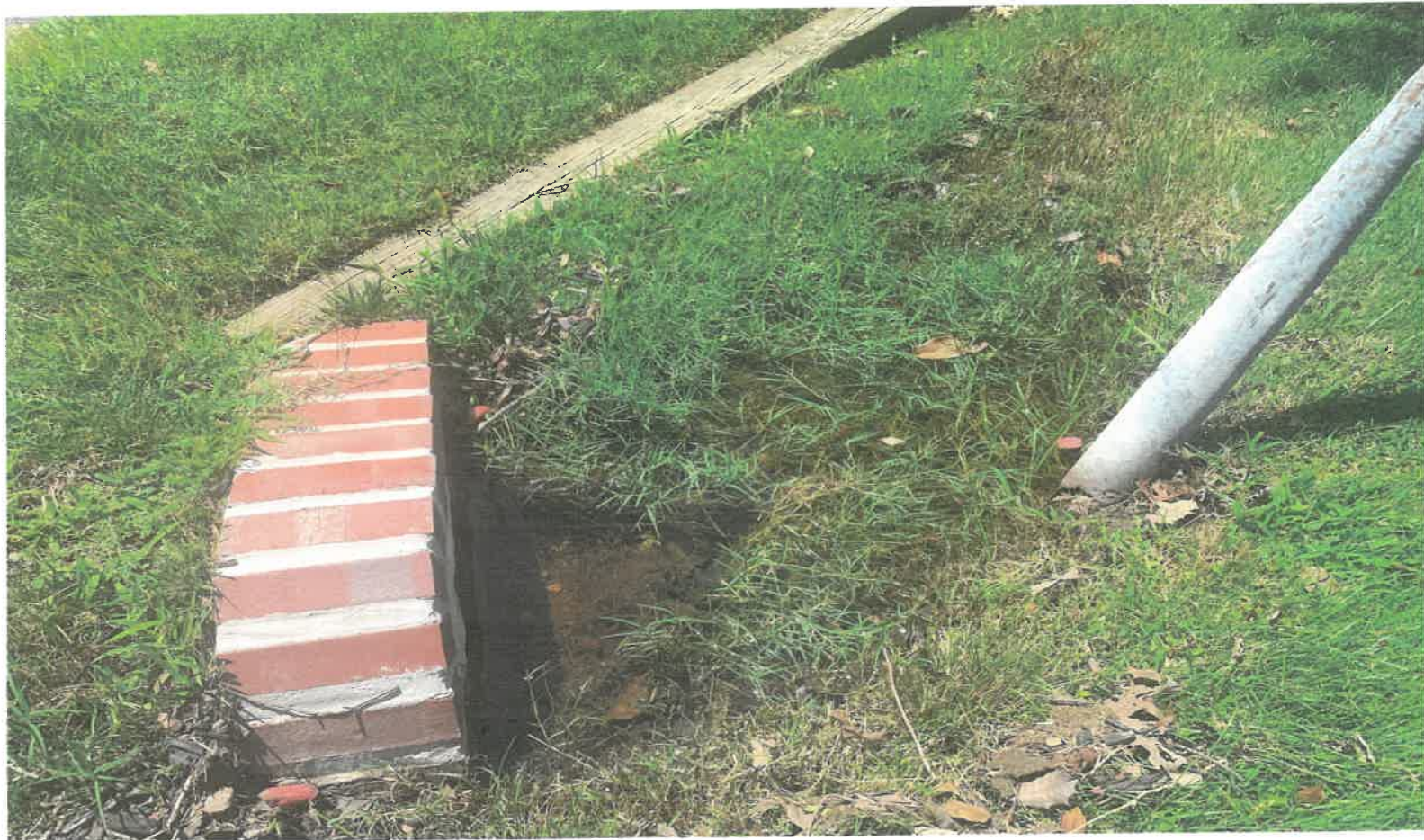
Existing RCP Storm Drain Running Under Cedar Drive
