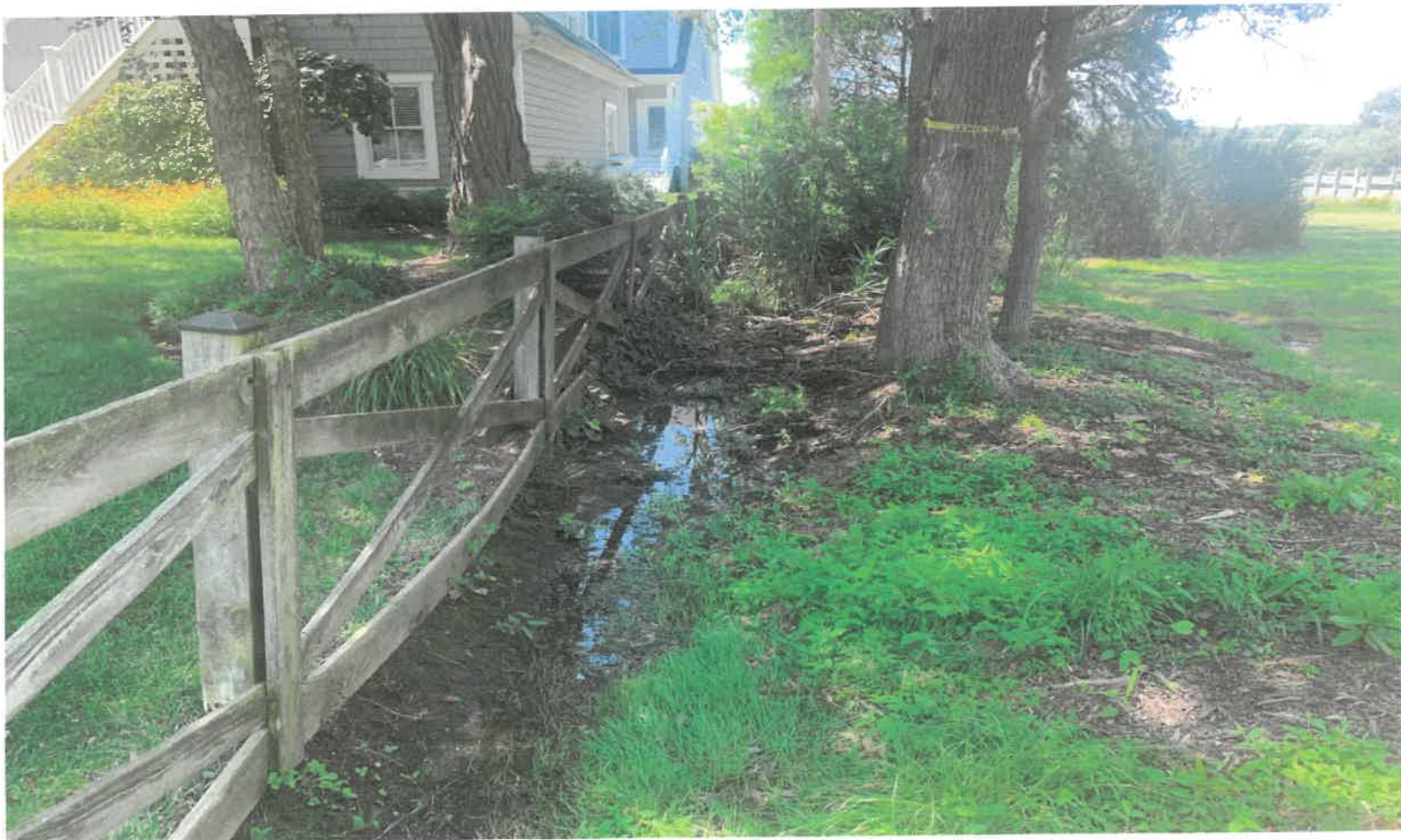
Drainage Swale Heading to Existing Sump Condition
