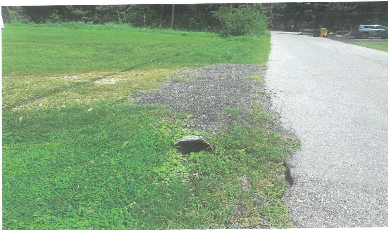
Existing 12" Culvert Pipe Running Under Existing Drive
