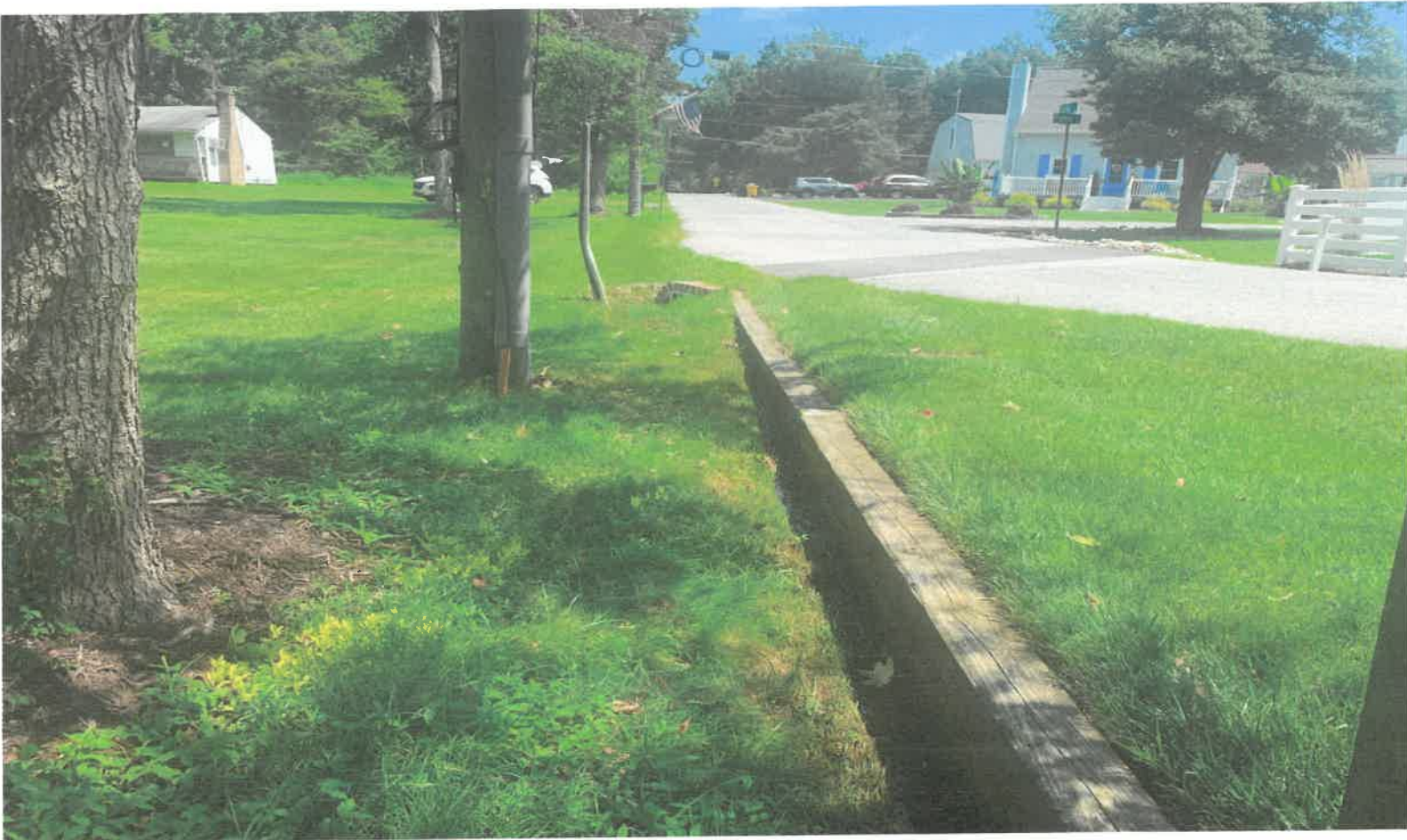
Existing Drainage Swale Flowpath Abutting Existing Retaining Wall
