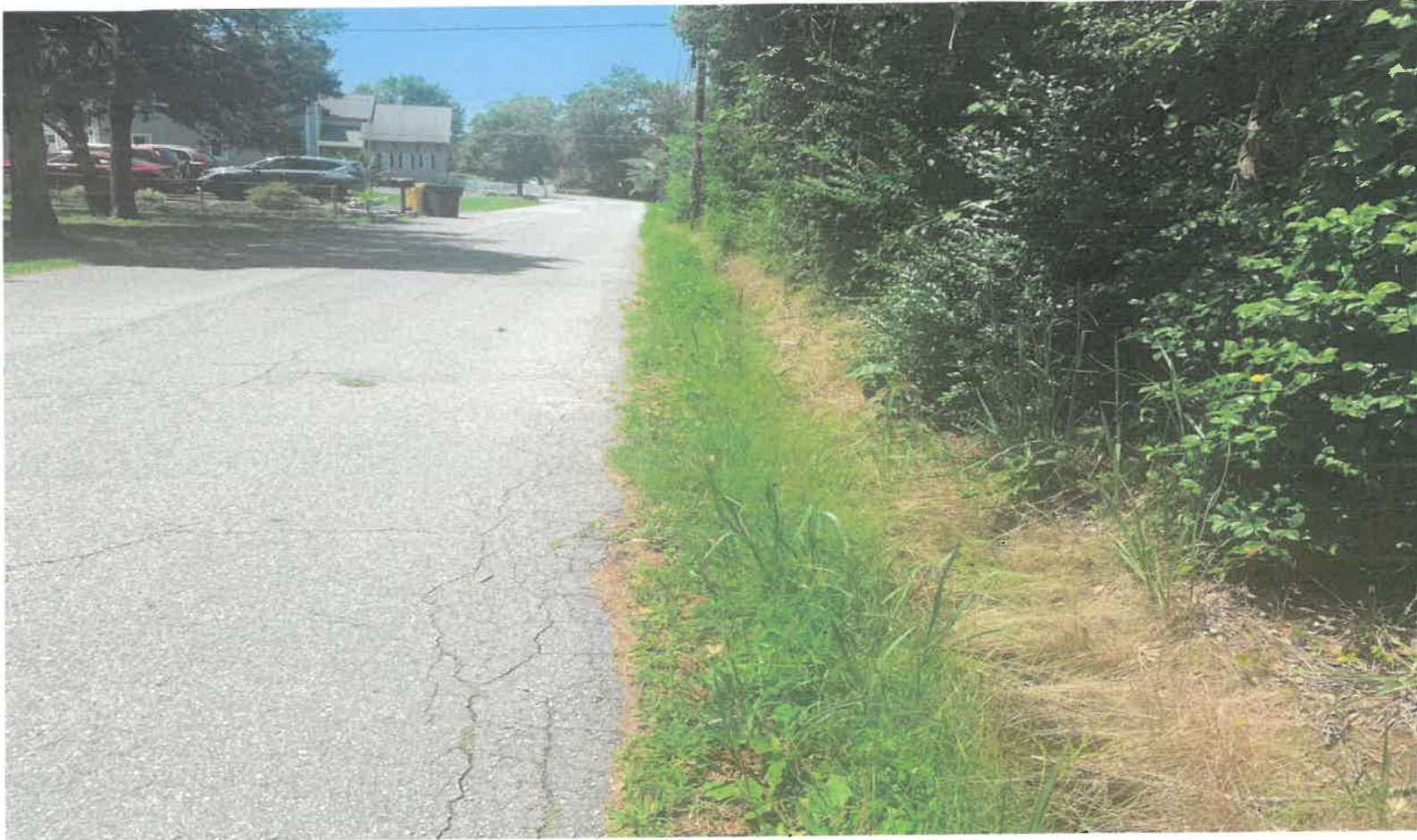
Existing Drainage Swale Along Cedar Drive
