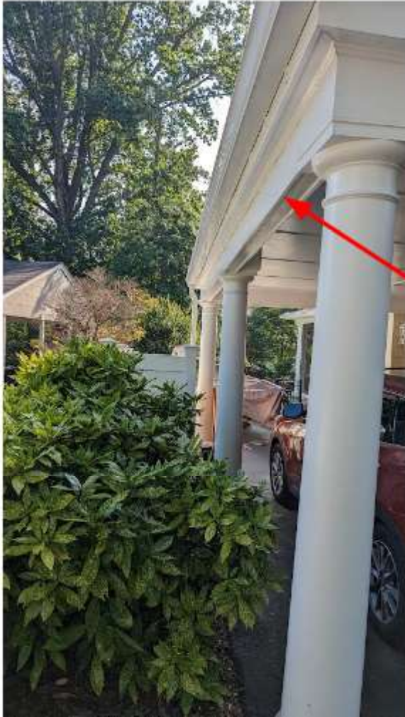
Figure 3: Existing framing is located on the exterior portion of columns. Walls will be constructed to this framing structure.
