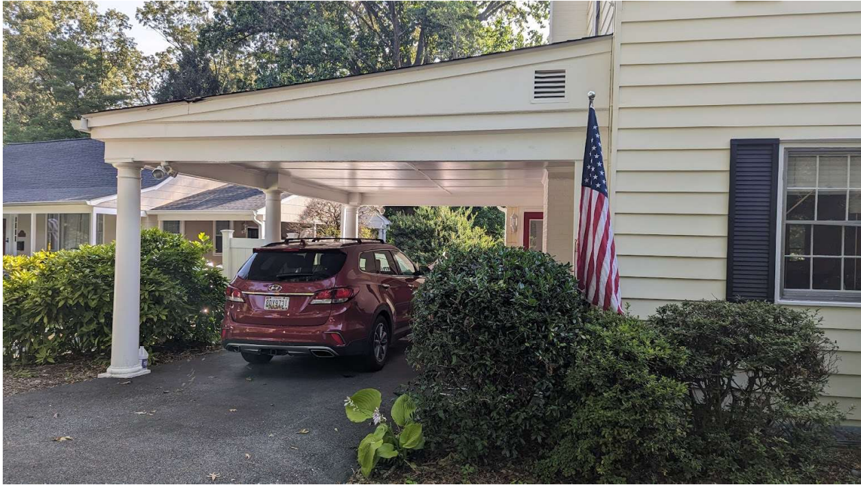
Figure 1: Carport showing existing columns and framing
