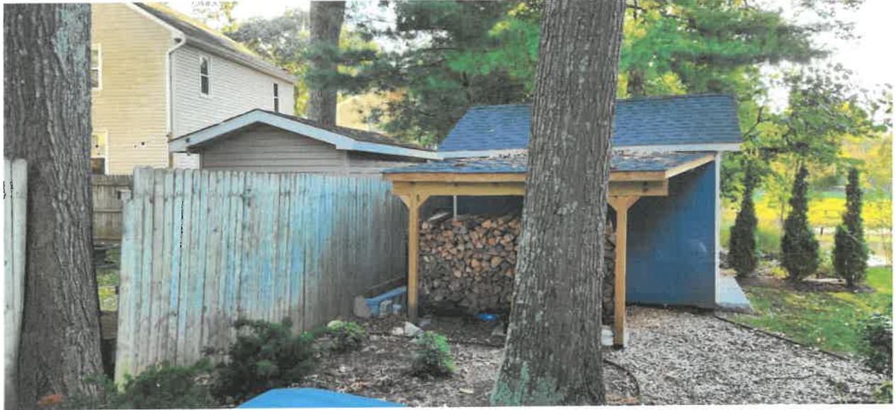
Figure 4 Side View of Sheds (Lot 11 Shed on left)
