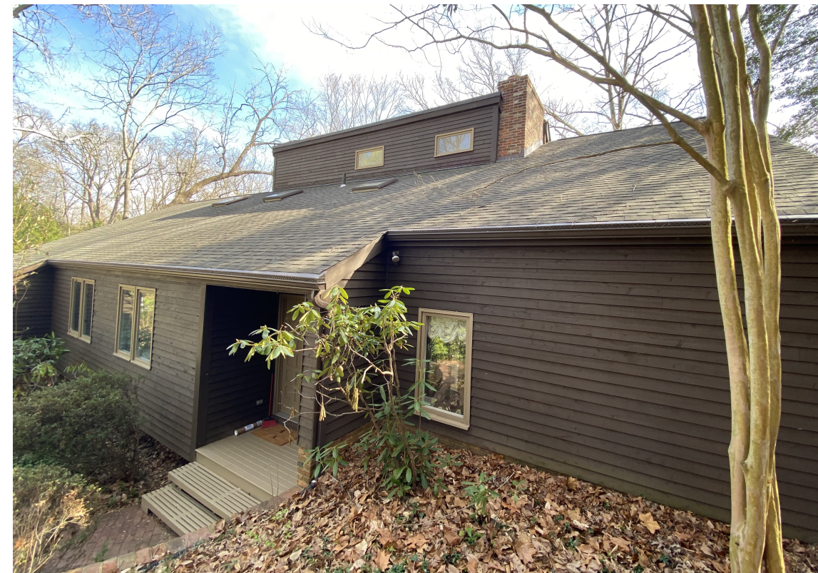
View of Existing Entry
