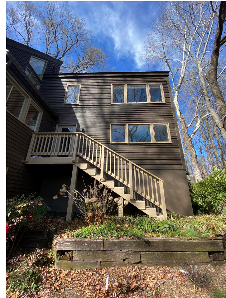
Rear of Garage - Waterside
