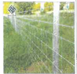
PAGE WIRE FENCE DETAIL 6.6 FT HIGH WELDED WIRE FENCE SUPPORTED BY A COMBINATION OF STEEL FENCE POSTS AND PRESSURE TREATED WOOD END AND CORNER POSTS
