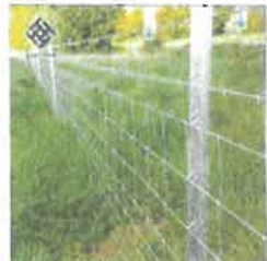
PAGE WIRE FENCE DETAIL 6.6 FT HIGH WELDED WIRE FENCE SUPPORTED BY A COMBINATION OF STEEL FENCE POSTS AND PRESSURE TREATED WOOD END AND CORNER POSTS
