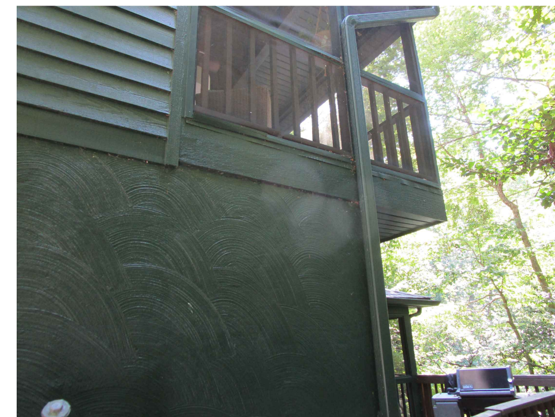
Existing First Floor Screened Porch
