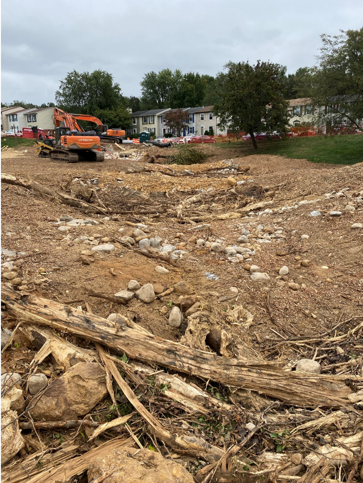
Figure B-16: Pond 1330 Retrofit (Anne Arundel County)
