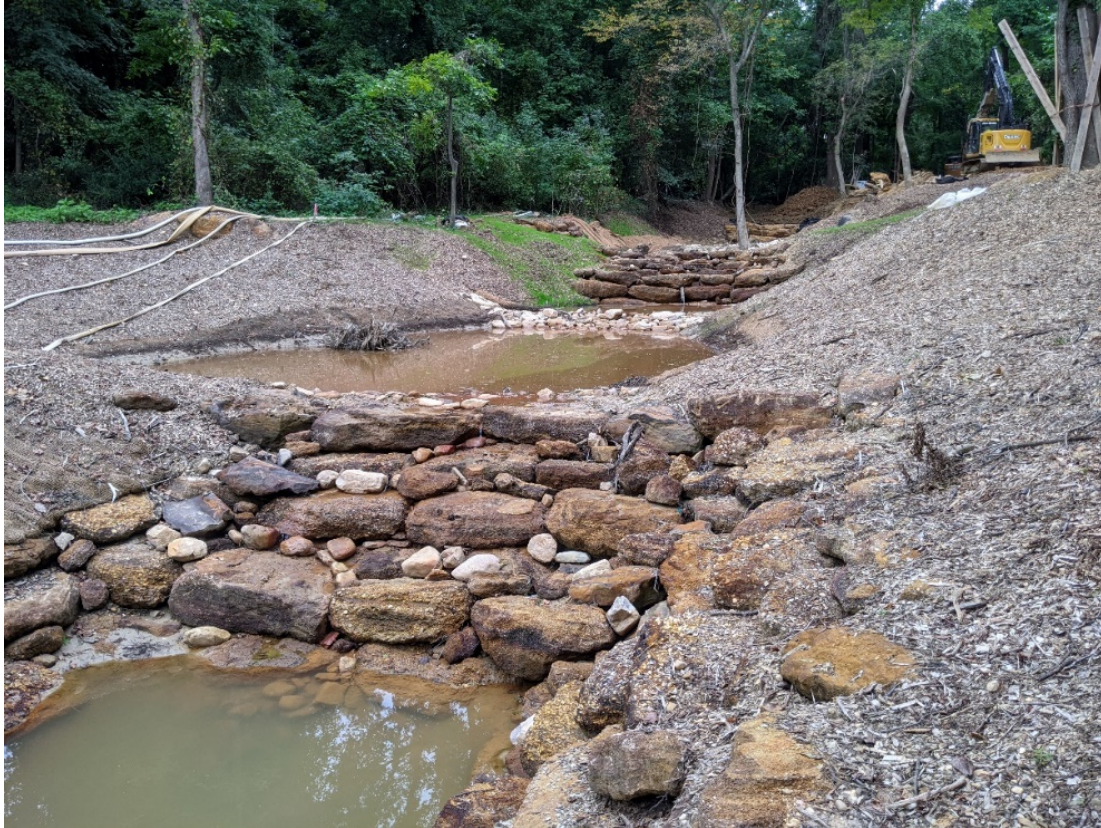
Figure 6: Cascade weirs during construction (Washington, DC)
