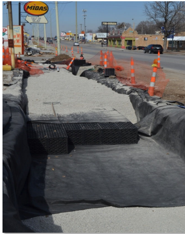
Storage Under Porous Pavers
