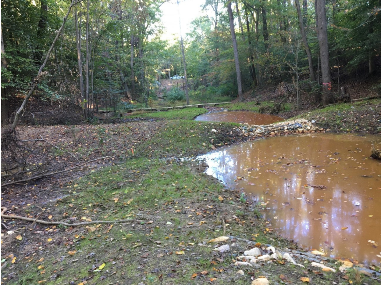
Figure 5: Riffle weir with berm (Forked Creek, Anne Arundel County)
