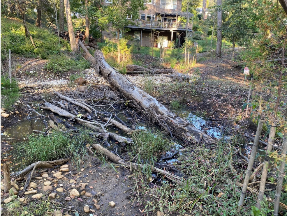
Figure B-8: Woody debris placement in a pool at Winchester SPSC (Anne Arundel County)
