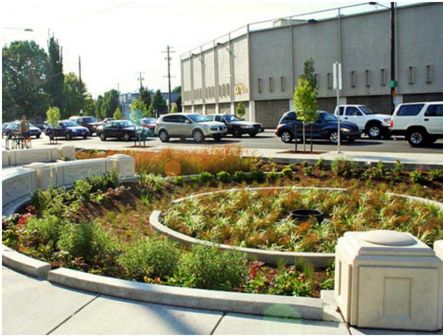
Figure 7: Multi-Functional Example: Depressed Roundabout with Bioretention
