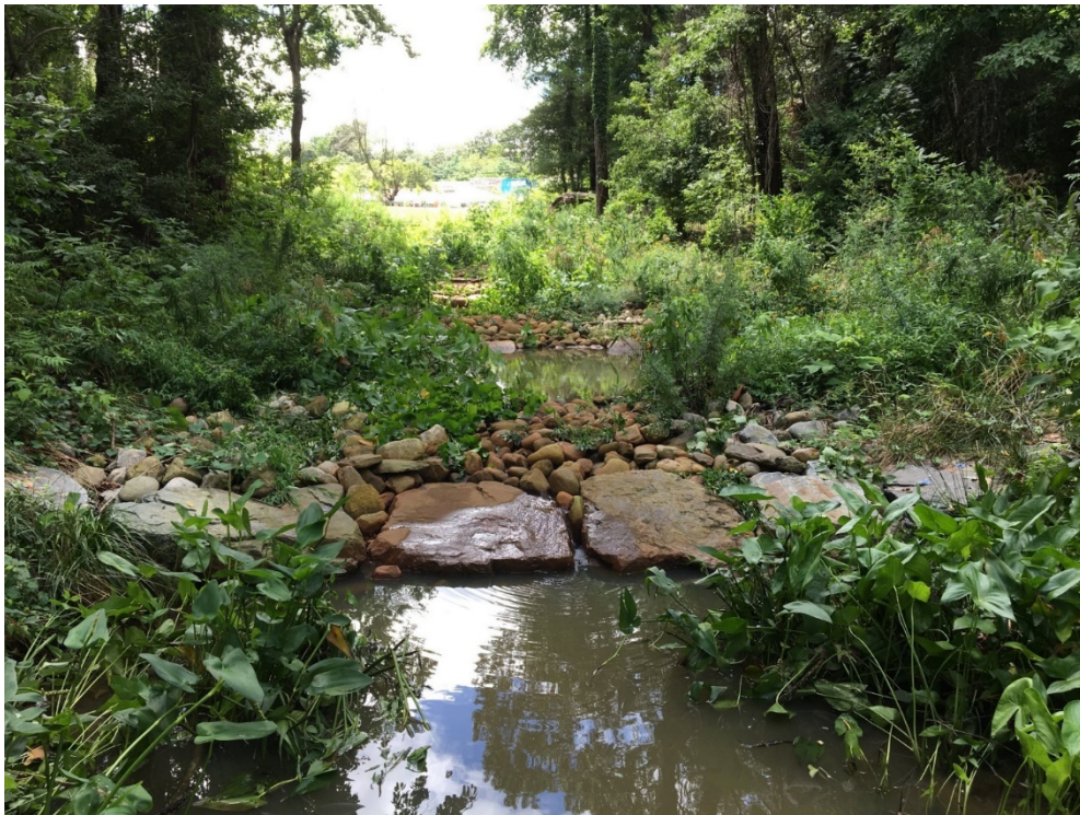
Figure B-3: Cape St. Claire Park SPSC – Magothy River Watershed (Anne Arundel County)
