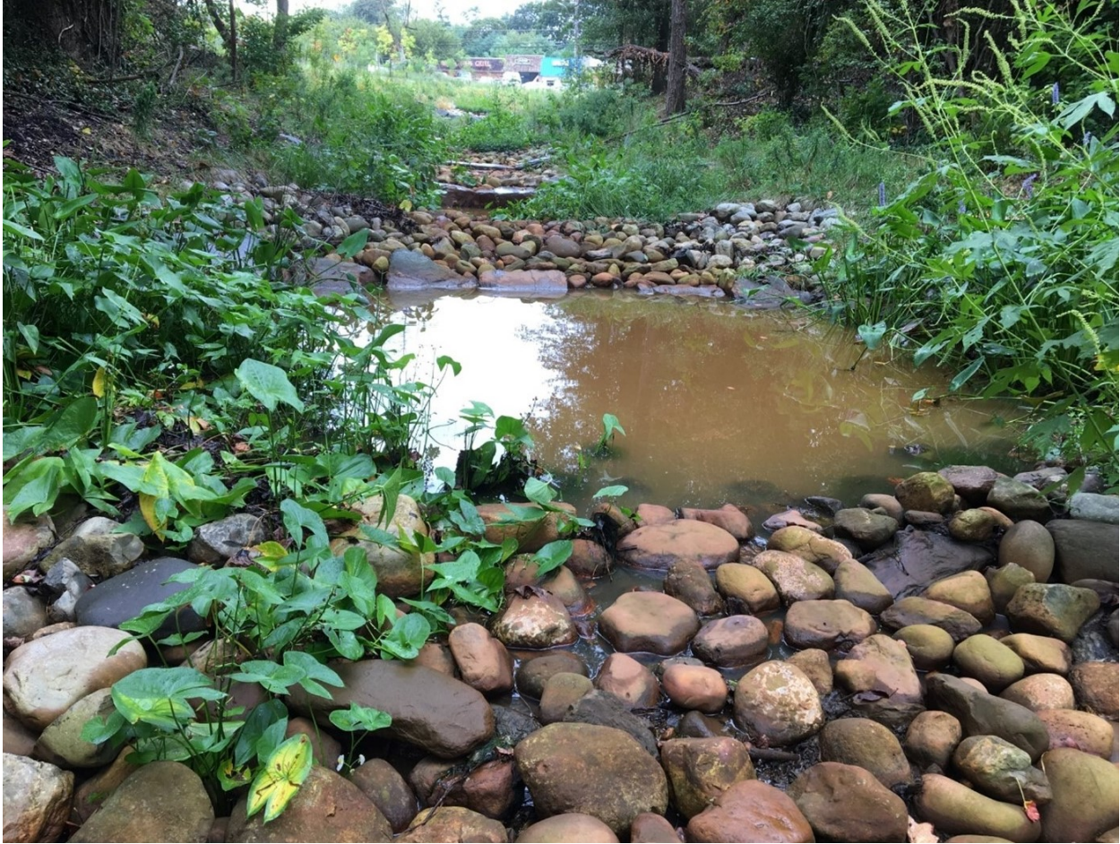
Figure 2: Riffle weir and pool sequence (Cape St. Claire SPSC)
