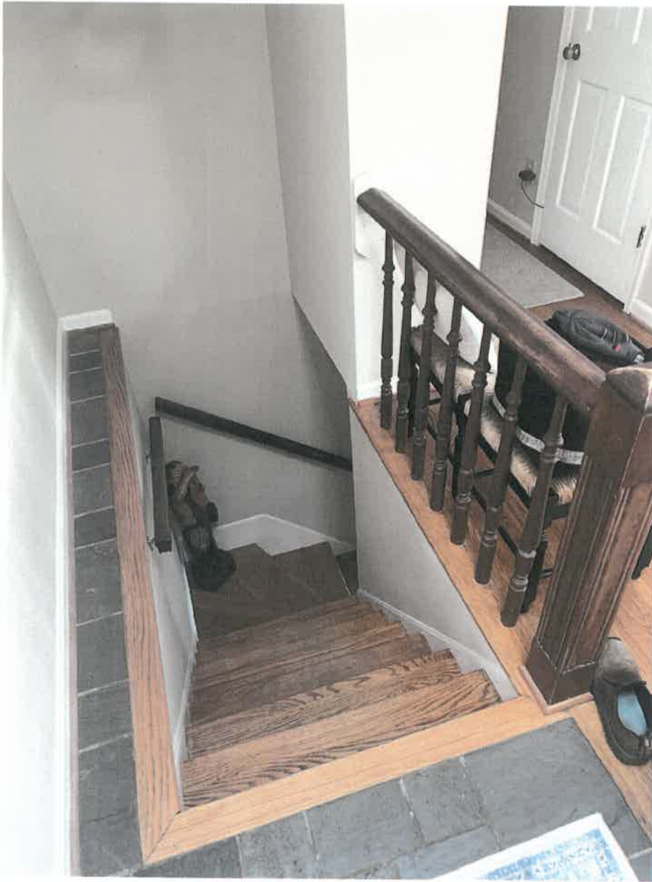
Existing Interior Staircase
