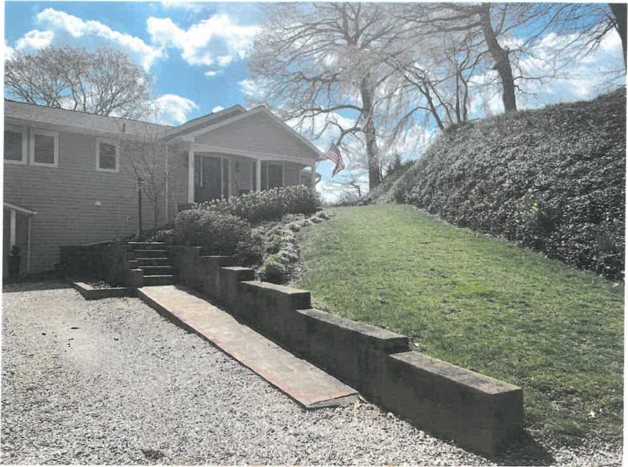
Existing Exterior Staircase
