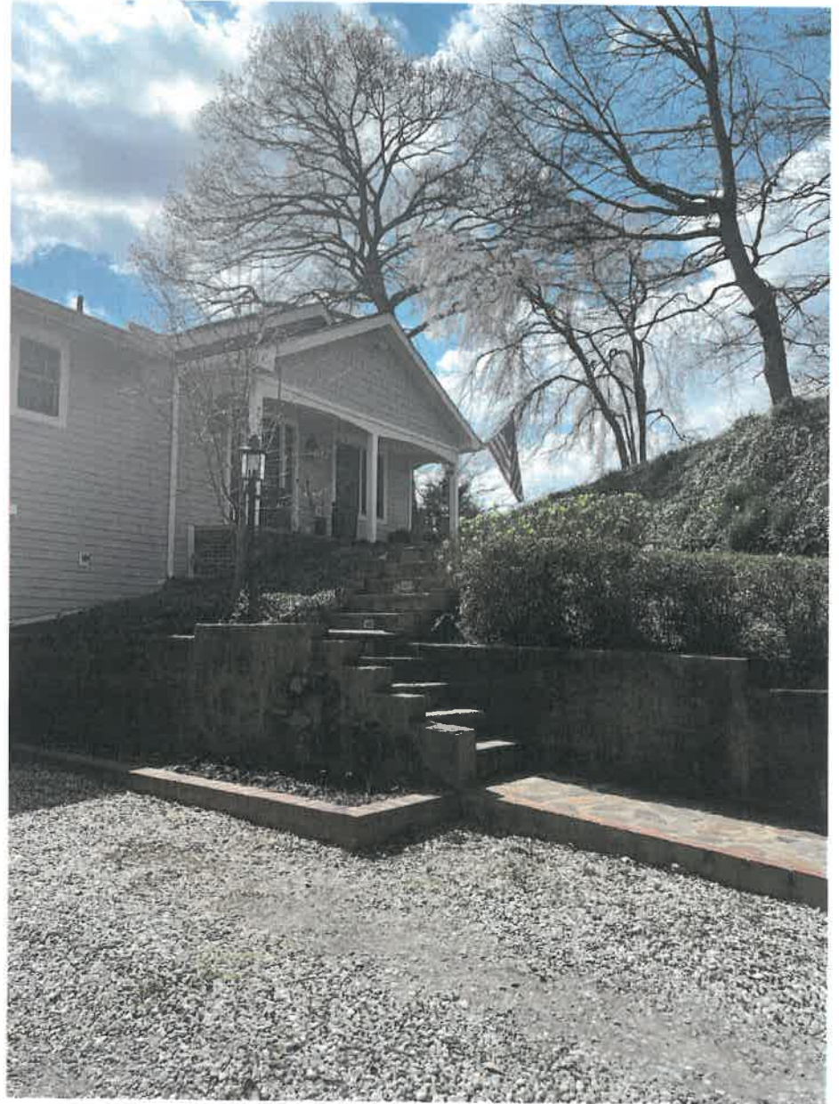
Existing Exterior Staircase
