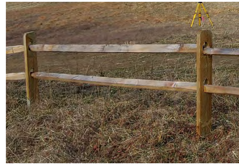
EXISTING 2-RAIL WOOD FENCE
