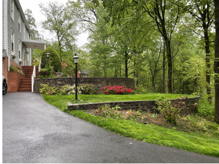
④ VIEW OF FRONT RETAINING WALLS
