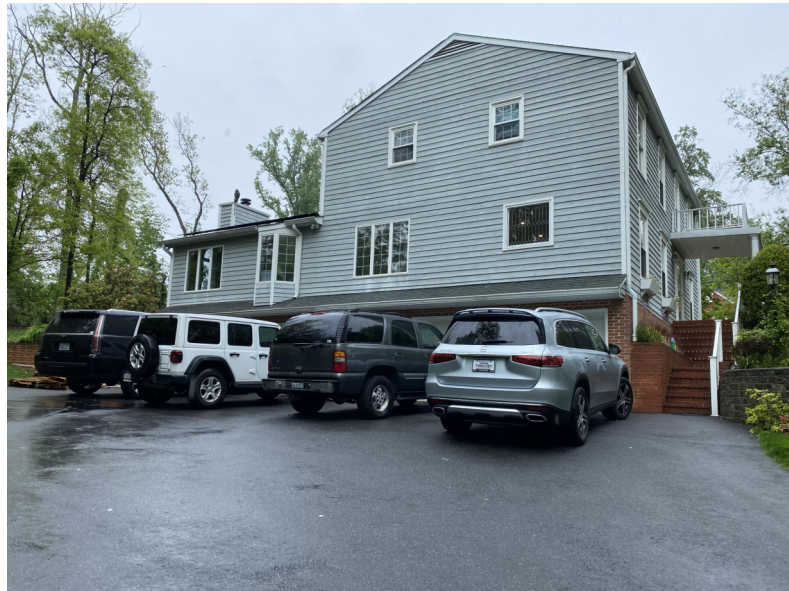
⑤ VIEW FROM EAST
