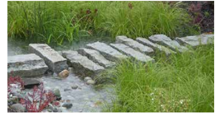
Weir Walls help slow stormwater and create artistic moments in the landscape
