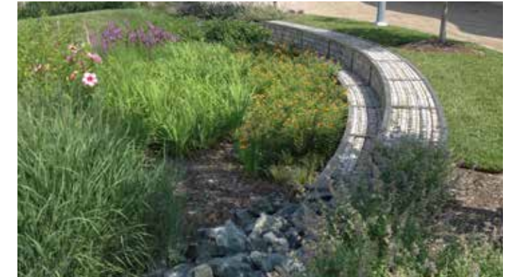
Rain Gardens - Gabion walls use natural materials that blend with the landscape and provide habitat for fauna.
