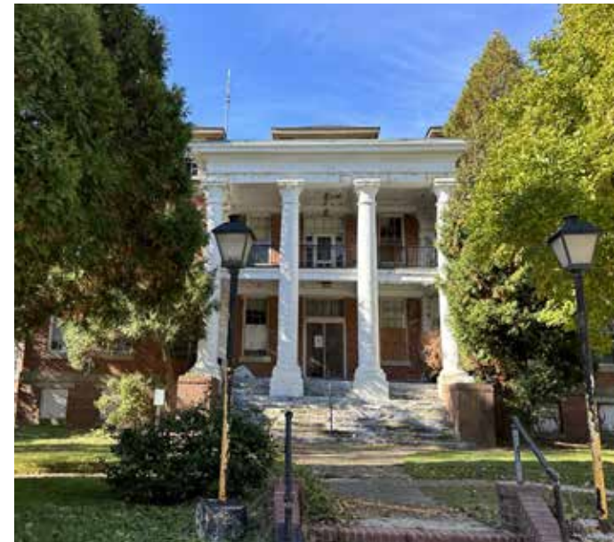
Admin Building - source: Design Collective
