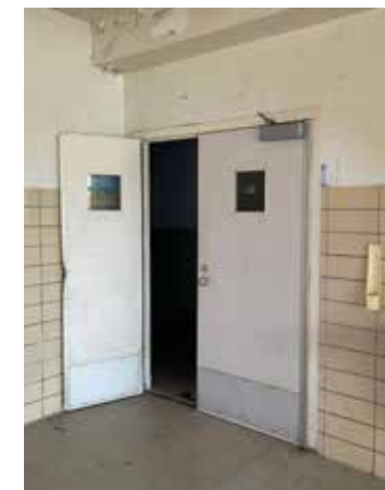
Meyer Building | Credit: EHT Tracerics
