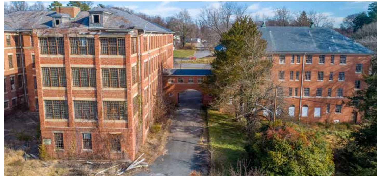
Existing Conditions - view of Admin Building and Nurse's Building looking east Credit: Anne Arundel County; Chesapeake Aerial Photography
