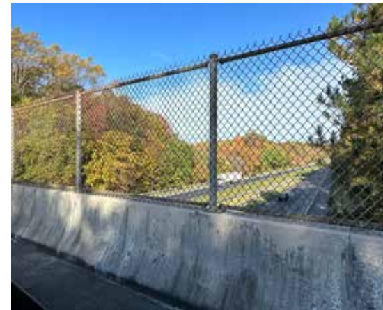
Bridge over I-97 - source: Design Collective
