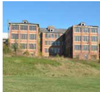
Laundry Building | Credit: DCI
