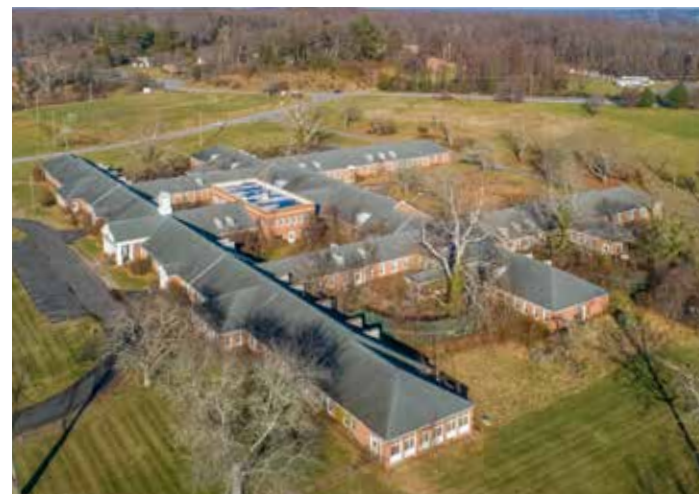
Meyer Building - Aerial View - December 2023 - source: Chesapeake Aerial Photography
