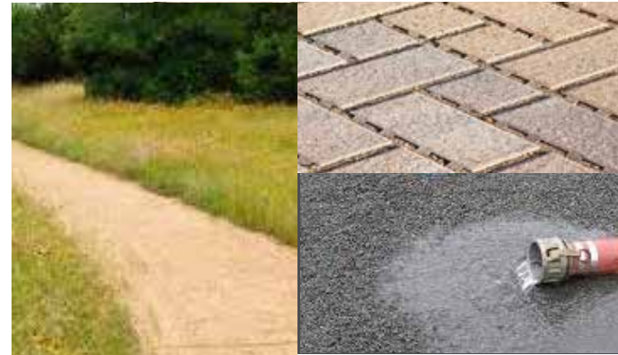
Permeable Paving - Alternative paving options such as unit pavers, porous concrete, porous asphalt reduce stormwater runoff
