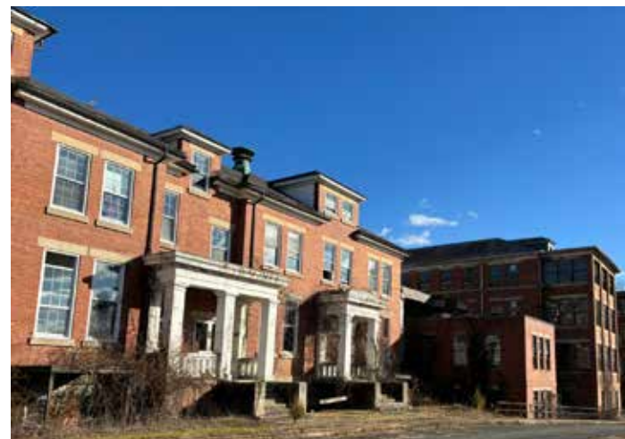
“B” Building - View of Rear Elevation - November 2023 - source: Design Collective
