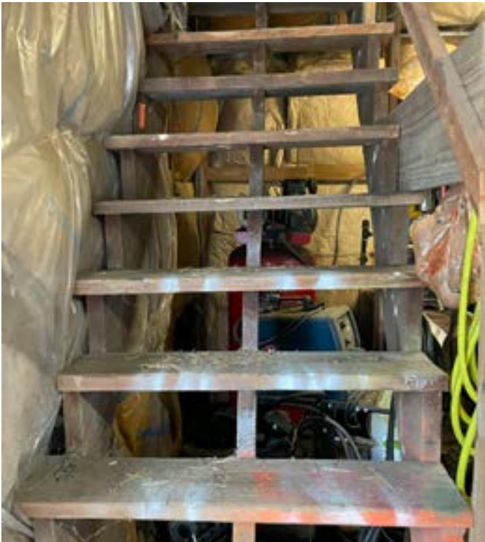
Figure 21. Existing stairs inside the barn Source: AECOM
