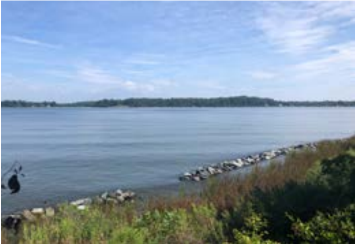
Figure 11. Shoreline protection/rip-rap Source: AECOM
