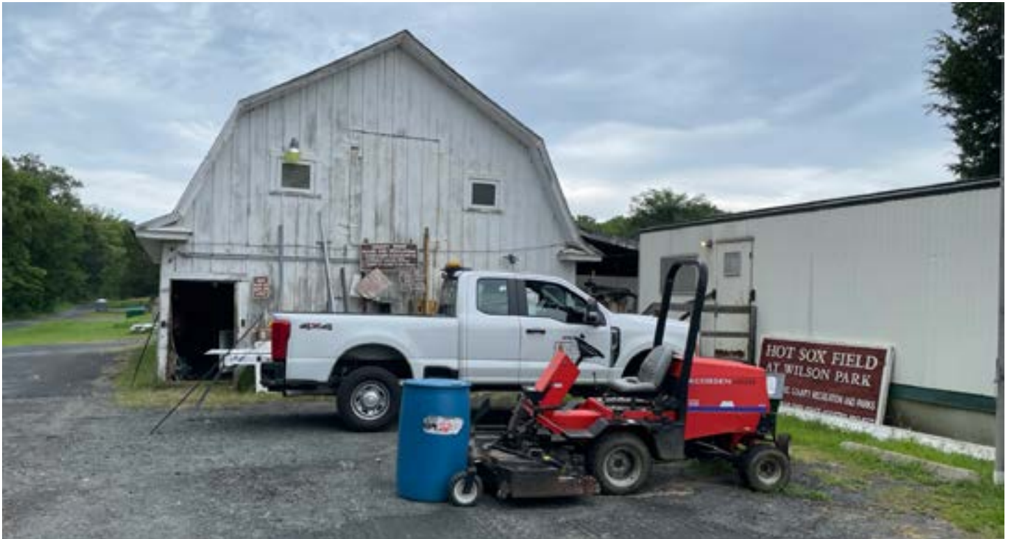
Figure 18. Existing barn and maintenance trailer
