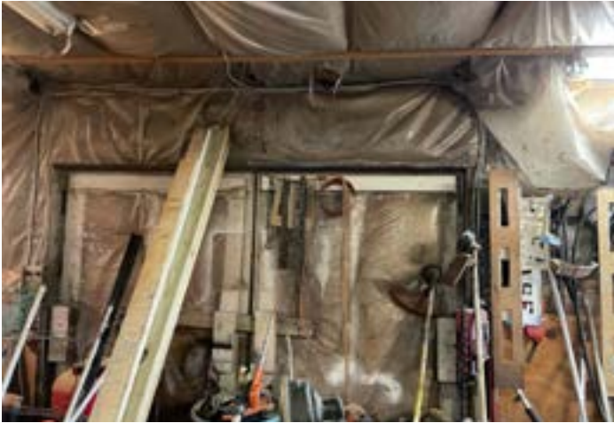
Figure 19. Interior walls and ceiling Source: AECOM
