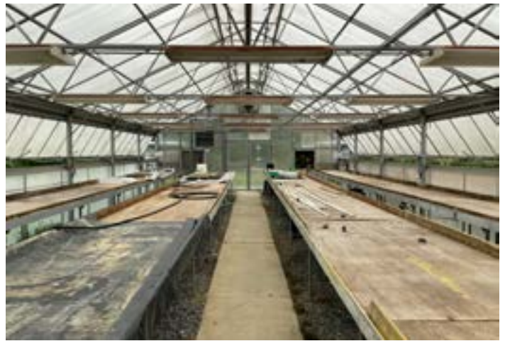
Figure 23. Interior of greenhouse
