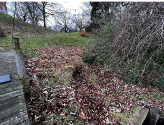
Photo 12 – Developing head cut at the shoreline
