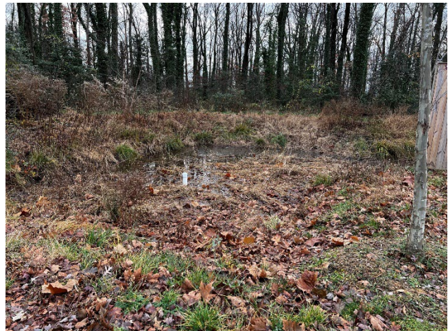
Photo 10 – Existing micro-bioretentation facility located southeast of the parking lot
