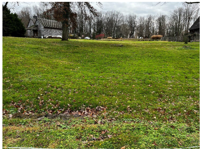
Photo 13 – Depressions in open space area
