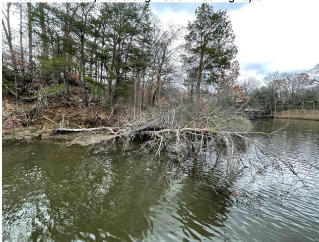
Photo 3 –Eroding Shoreline along Reach 2 on Almshouse Cove
