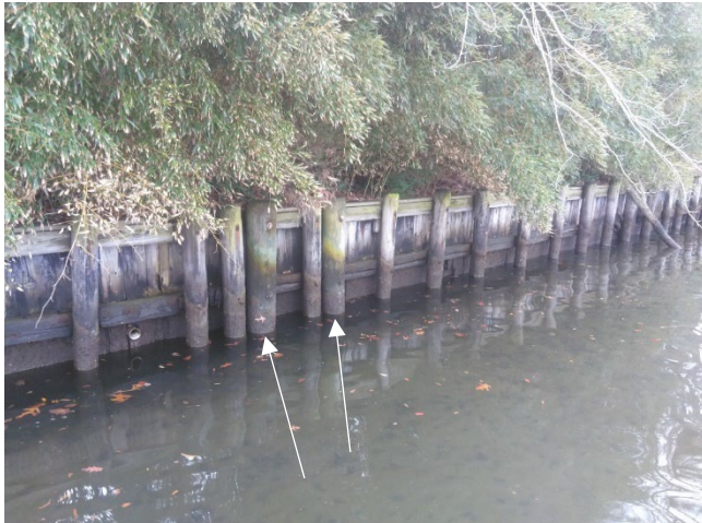
Photo 1 – Added piles along Reach 1 during repair
