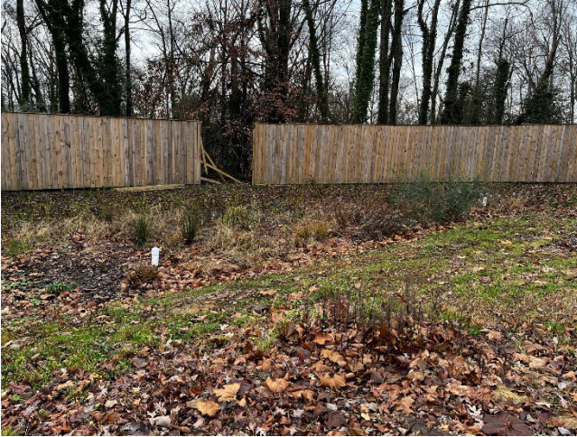
Photo 11 – Existing micro-bioretenion located south of the parking lot
