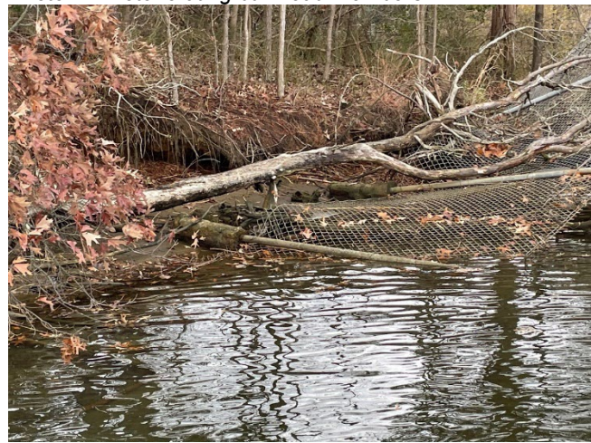
Photo 4 – Undercutting and fallen fence and trees on Almshouse Cove
