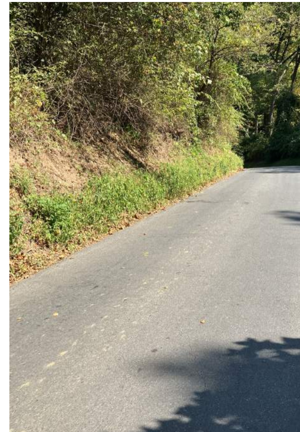
Figure 83. Existing Honeysuckle Road
