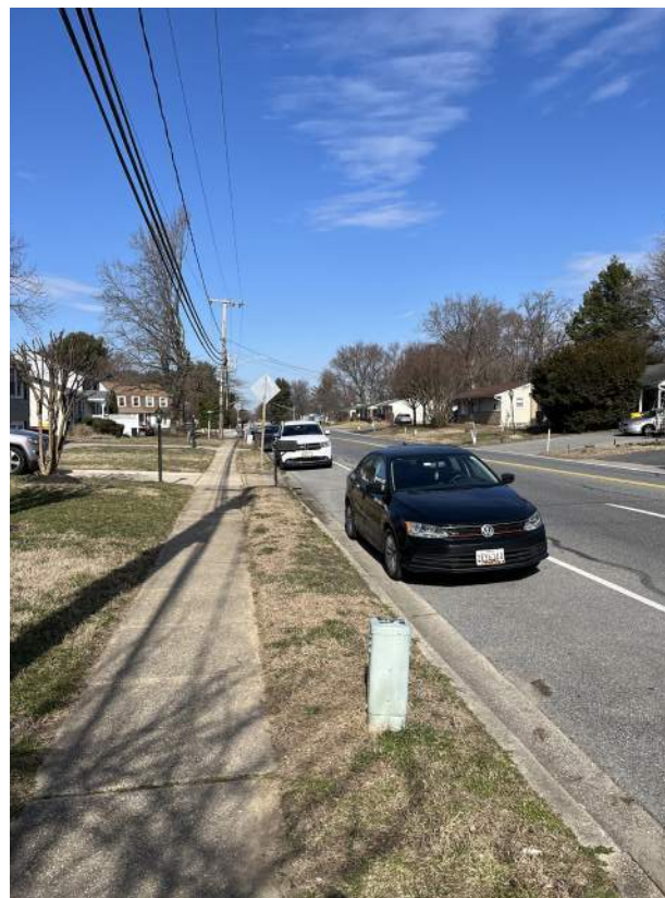
Figure 41. Existing Mago Vista Road parking
