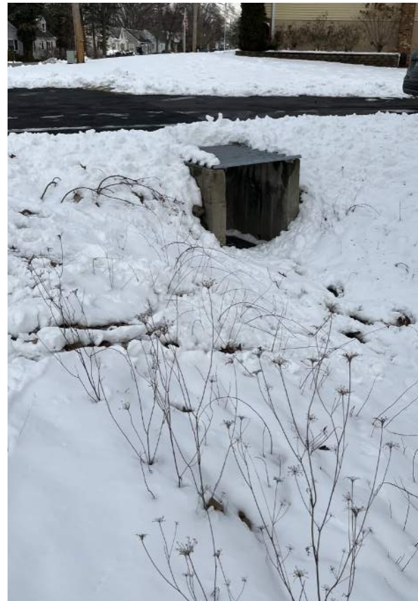
Figure 62. Existing drainage structures to be modified
