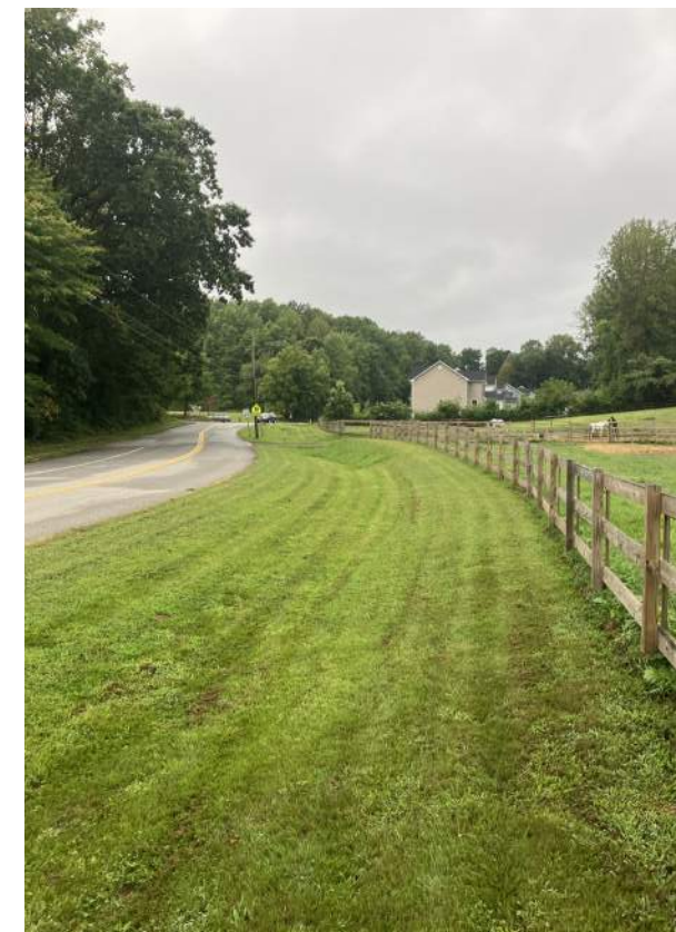
Figure 59. Existing shoulder along Broadneck Road
