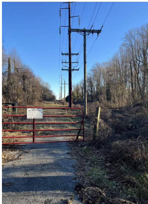
Figure 77. Existing BGE Power Line and future South Shore Trail Phase 3 Alignment
