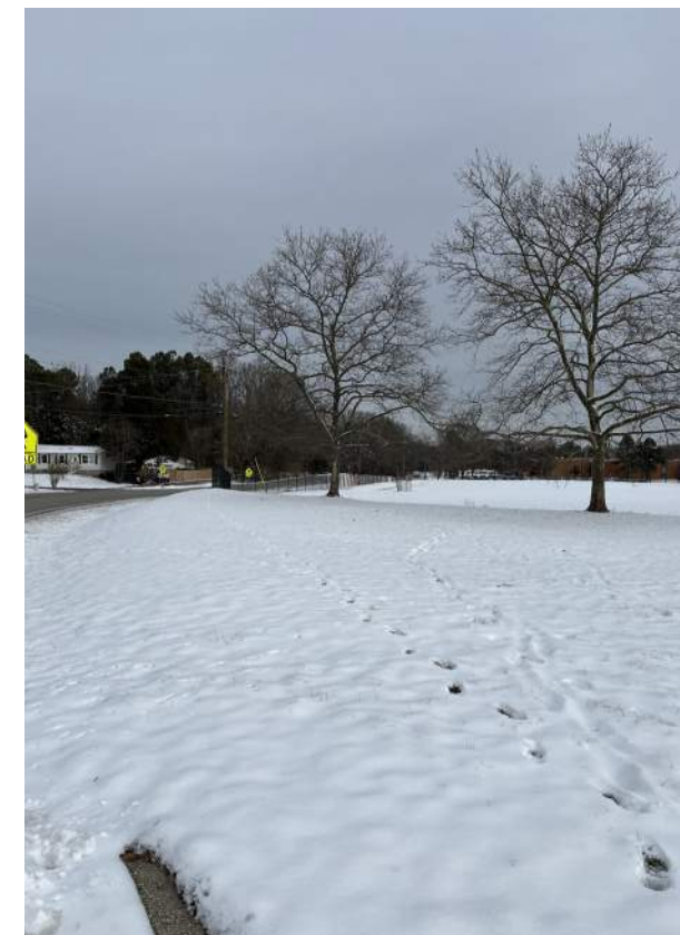
Figure 55. Peninsula Farm Road shoulder
