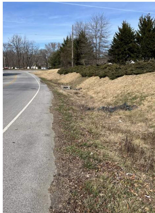
Figure 70. Crownsville Road drainage ditch
