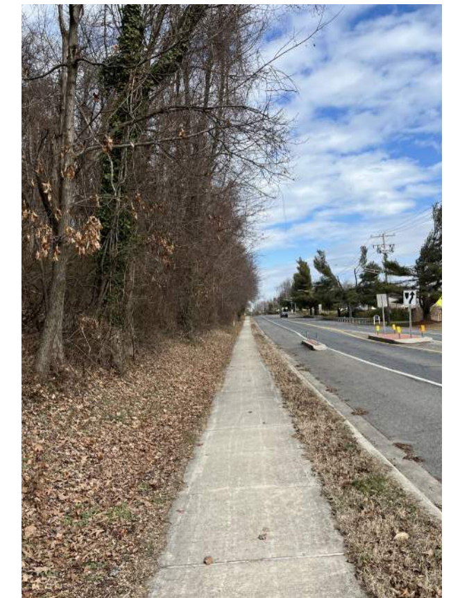
Figure 48. Shore Acres Road shoulder
