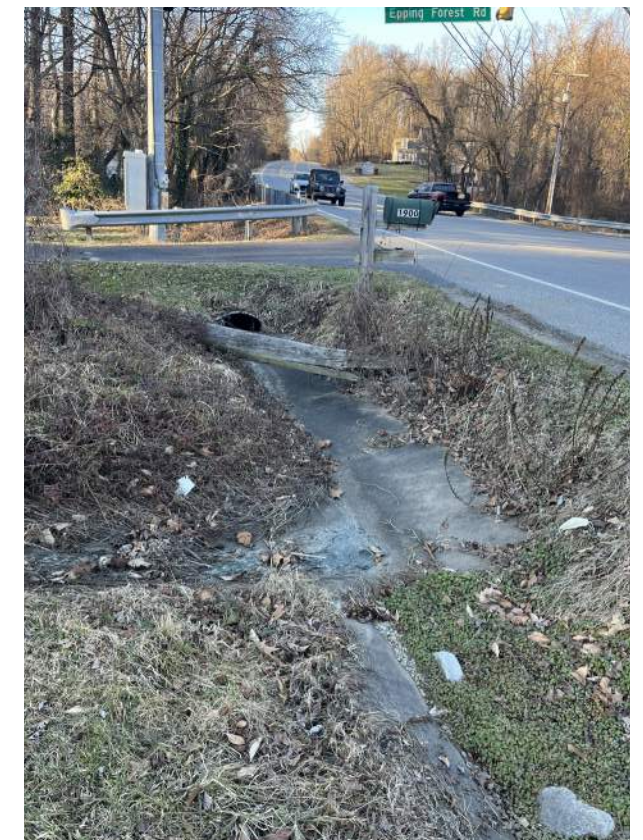
Figure 80. Drainage structures at Generals Highway and Epping Forest Road
