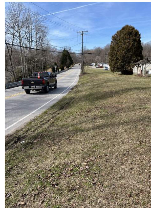
Figure 71. Crownsville Road shoulder
