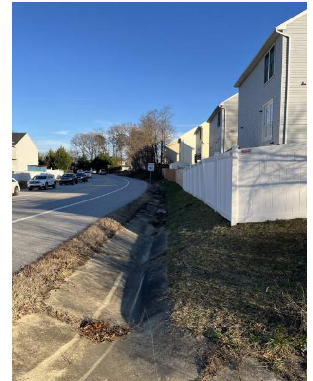
Figure 24. Existing open drainage ditch along Earleigh Heights Road
