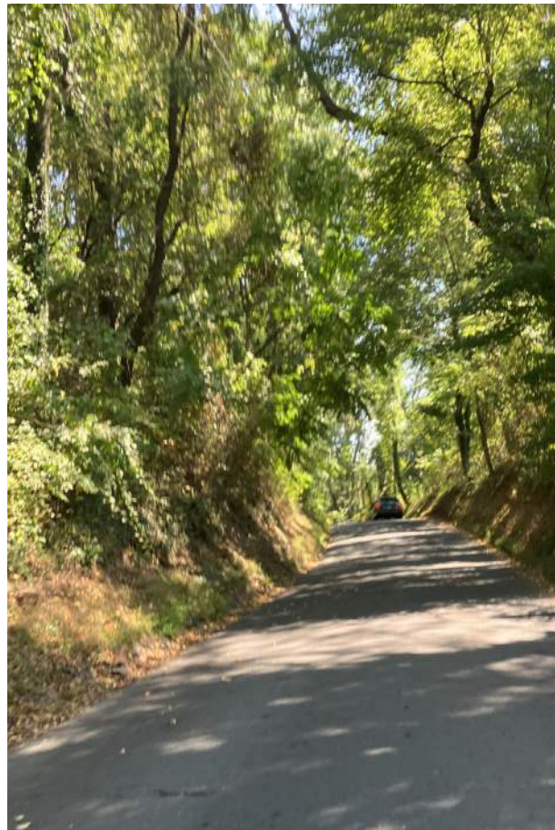
Figure 81. Existing Honeysuckle Road
