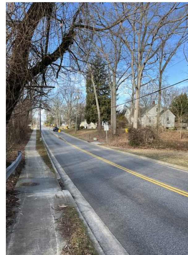
Figure 27. Existing Sidewalk along Pasadena Road
