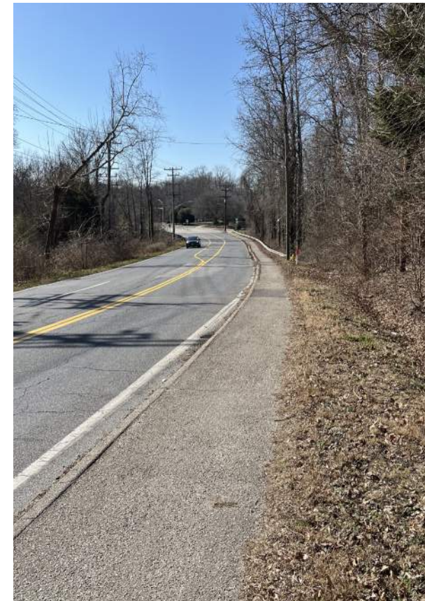
Figure 43. Jones Station Road shoulder
