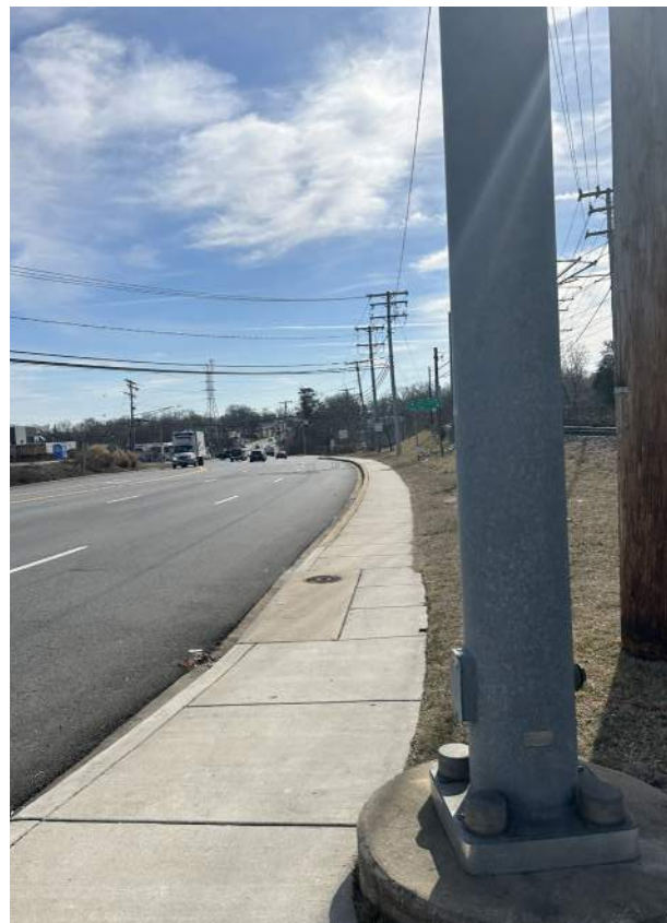
Figure 13. Exit from Cromwell Station Park & Ride looking Southeast along Dorsey Road. Existing traffic Signal Equipment
