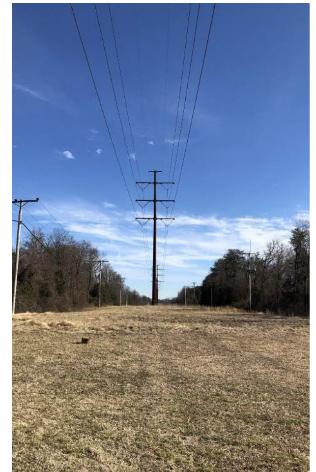
Figure 12. Foxbridge looking Northeast along existing BGE Right-of-Way
