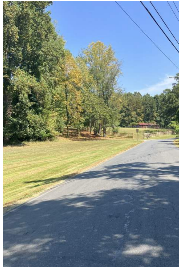
Figure 82. Existing Honeysuckle Road
