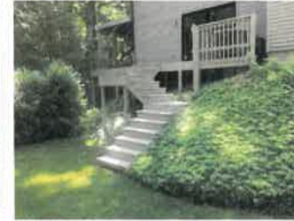
9. Side Yard Beveled Deck and Stairs - Looking to South East
