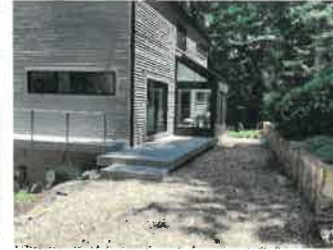
8. Upper Parking Area, Stone Retaining Wall, Entrance Deck and House - Looking to North East
