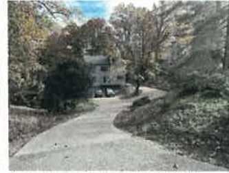
3. Driveway, Frontyard and Location of New Steps to Street and Front of House
