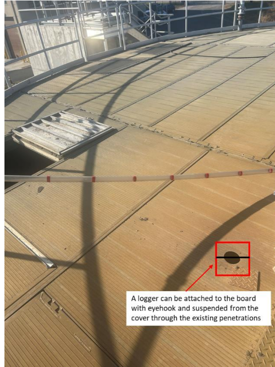
Figure 2-6 Gravity sludge thickener PPM monitor location
