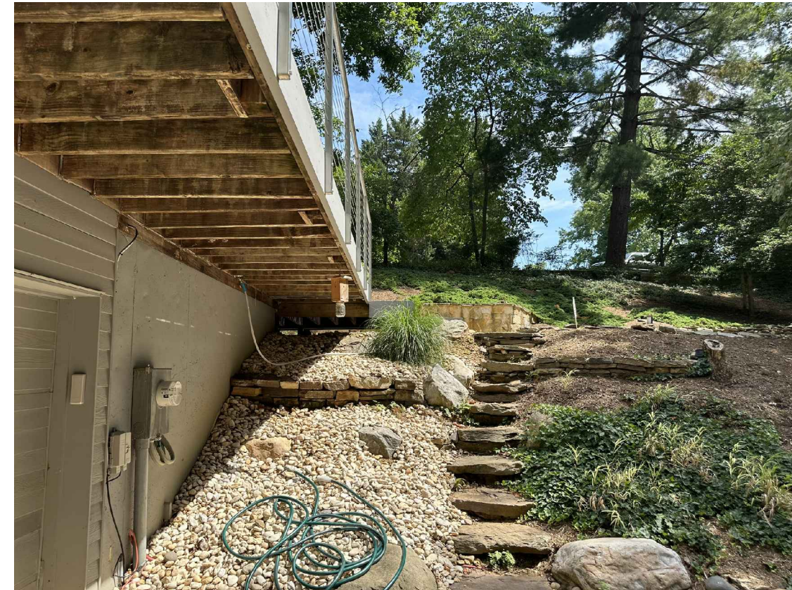
6. Boulder Stairs to Cantilevered Entrance Deck Adjacent to Garage Doors - Looking South
