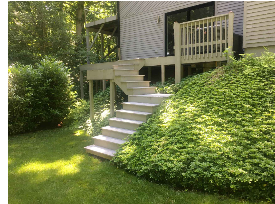
9. Side Yard Elevated Deck and Stairs - Looking to South East
