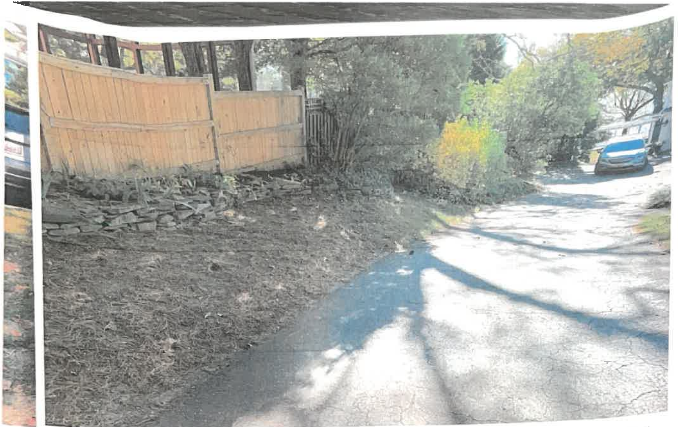
Photo Location #2 Looking Southwest Towards Existing Steep Slopes, Stable With Vegetation & Existing Flagstone Wall
