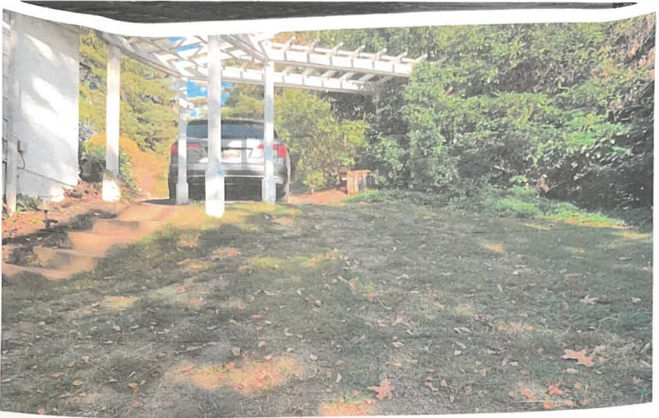
Photo Location #4 Looking Northeast Up Steep Slopes
