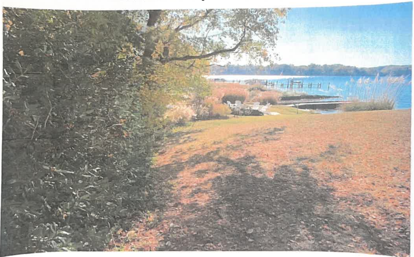
Photo Location #5 Looking South Across Steep Slopes, Area Stable With No Erosion Present
