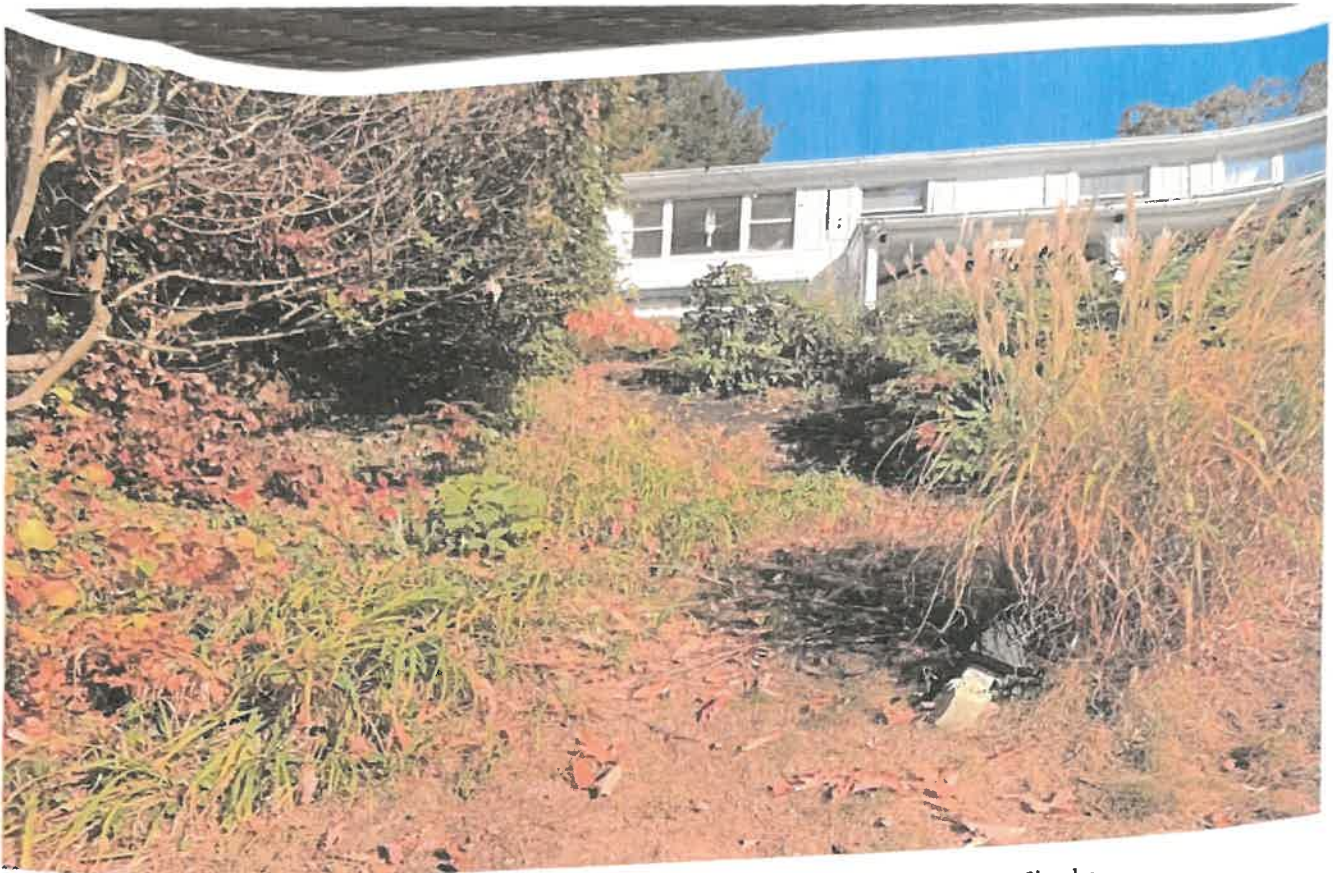
Photo Location #12 Looking East Up Slope, Area Stable With Ground Cover & Shrubs
