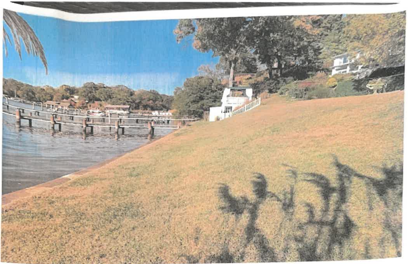
Photo Location #8 Looking North, Steep Slopes Stable With Lawn & No Erosion Present
