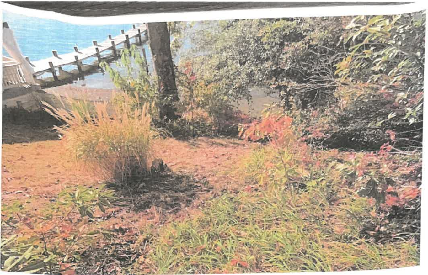
Photo Location #13 Looking West Down Slope, Area In Good Condition With No Erosion Present
