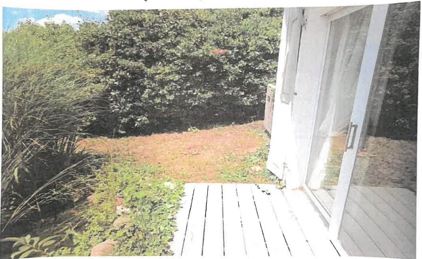
Photo Location #14 Looking North From Existing Wood Deck, Area Stable With No Erosion Present
