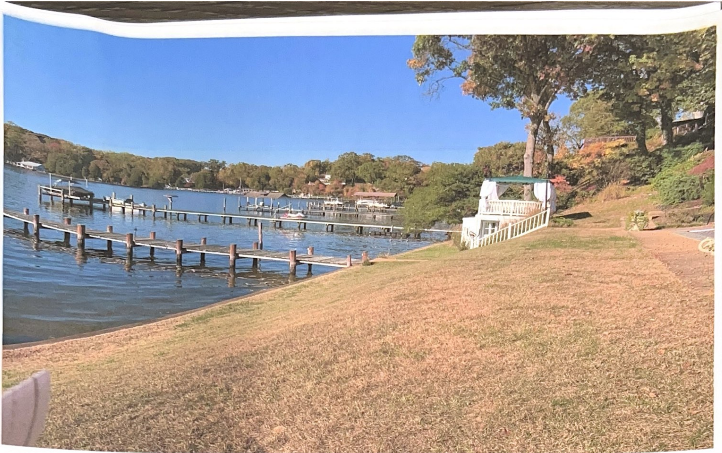
Photo Location #9 Looking Northwest From Top Of Slopes, Area Stable With Lawn In Good Condition
