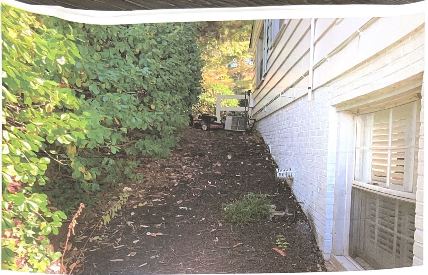
Photo Location #15 Looking East Up Existing Slope, Area Stable & In Good Condition
