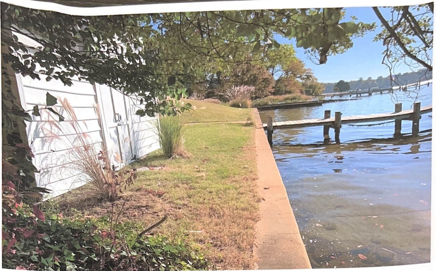
Photo Location #10 Looking Across Bulkhead Towards Toe Of Slope, Area Stable With No Erosion Or Sediment Present
