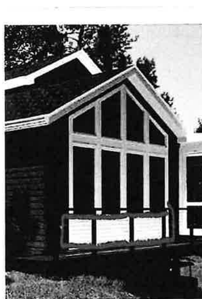
Area to be painted to match the siding
