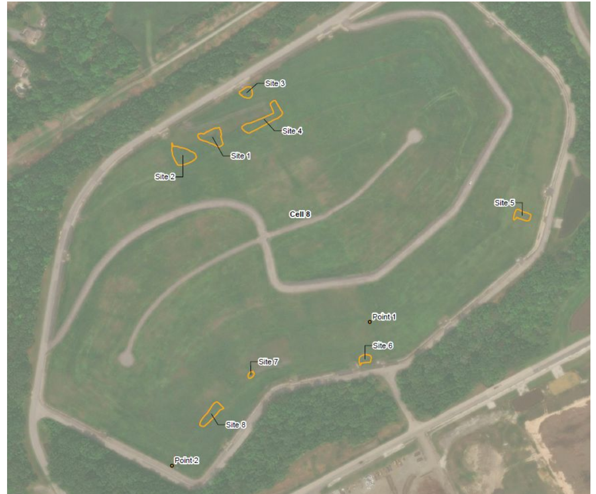
Cell 8 Repairs identified by EA Engineering (2024)
