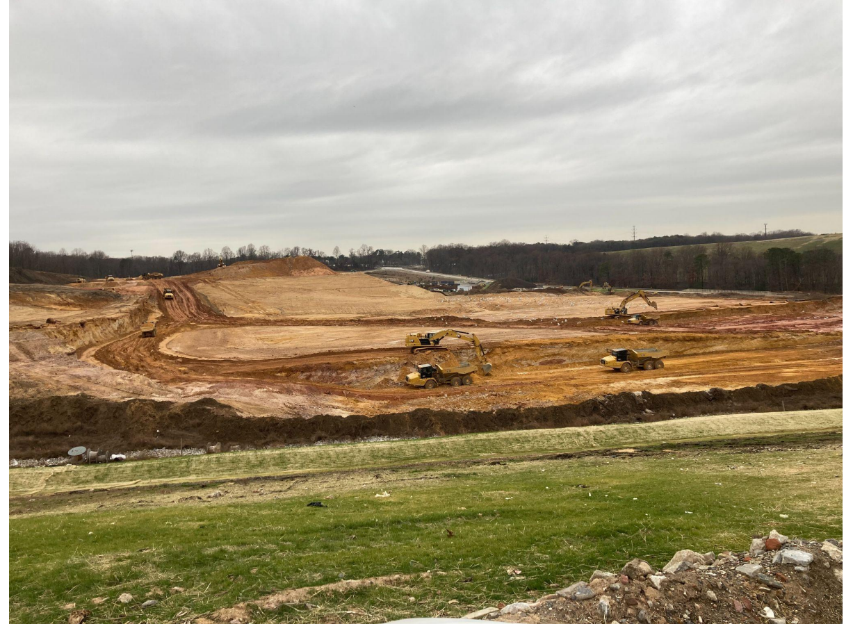
Subcell 9.3 Excavation Work (December 2024)
