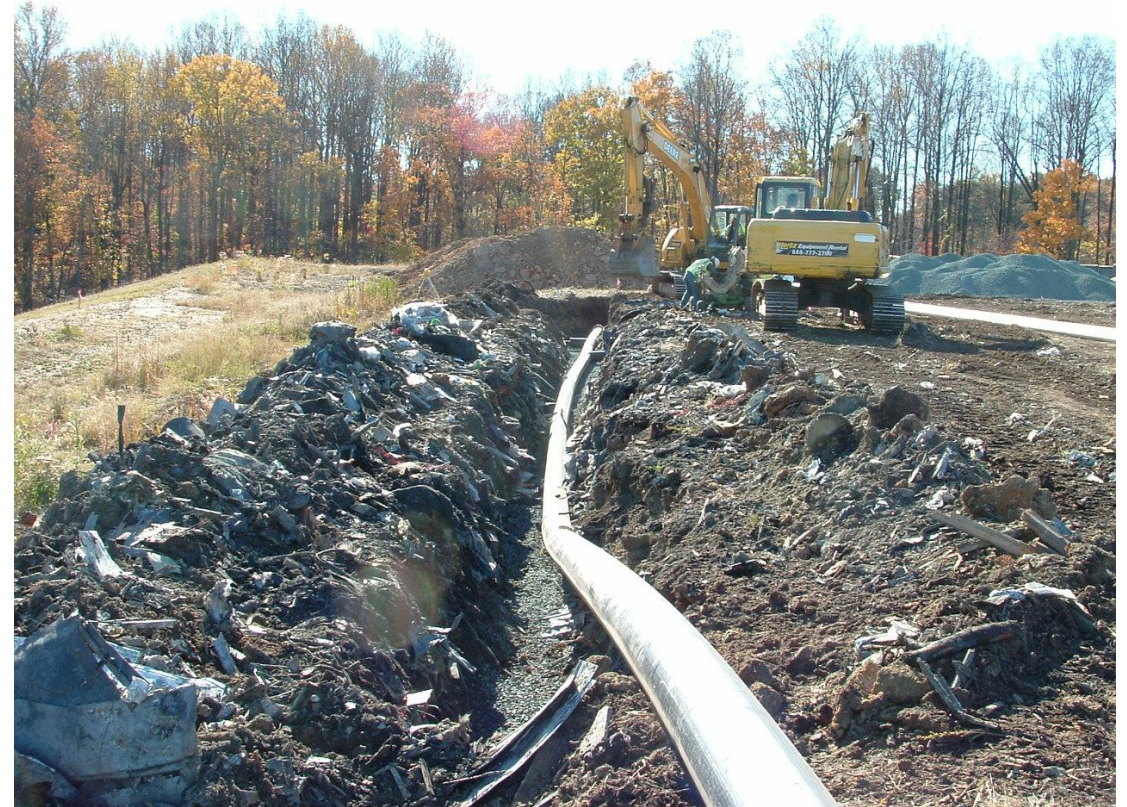
Temporary Gas Collection System Install Subcell 9.1
