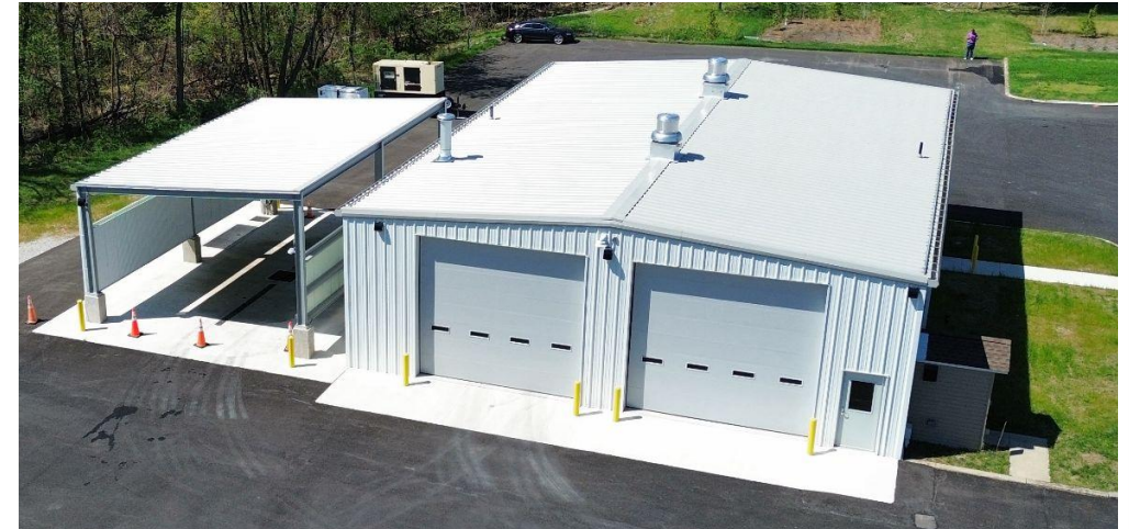
MLF Warehouse Renovation (2024)
