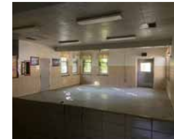
Meyer Building | Credit: EHT
