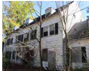
Superintendent's House | EHT
