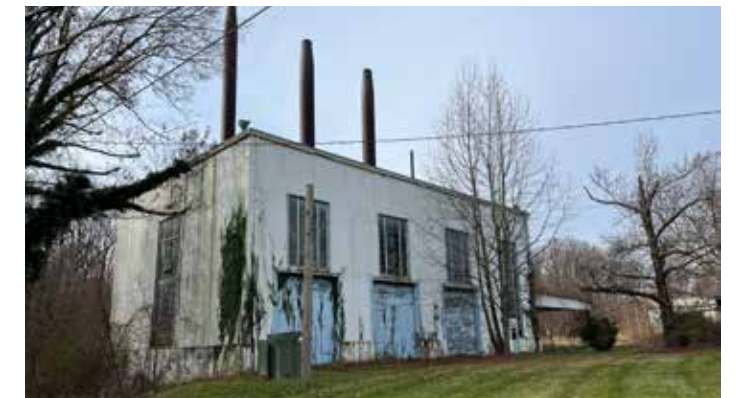
Boiler Plant - source: EHT Traceries
