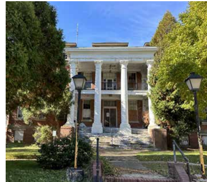
Admin Building - source: Design Collective
