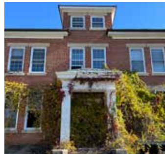
"B" Building | Credit: DCI
