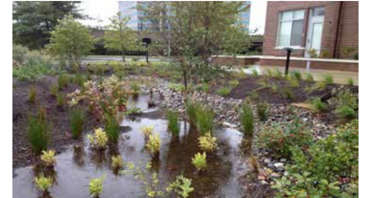
Rain Gardens - Natural depression in the landscape help capture, store, cleanse and infiltrate stormwater.
