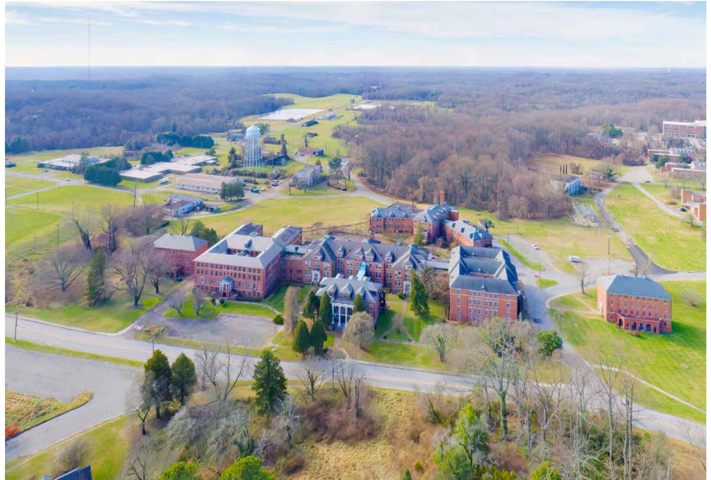
Existing Conditions - view from Crownsville Road looking West Credit: Anne Arundel County; Chesapeake Aerial Photography
