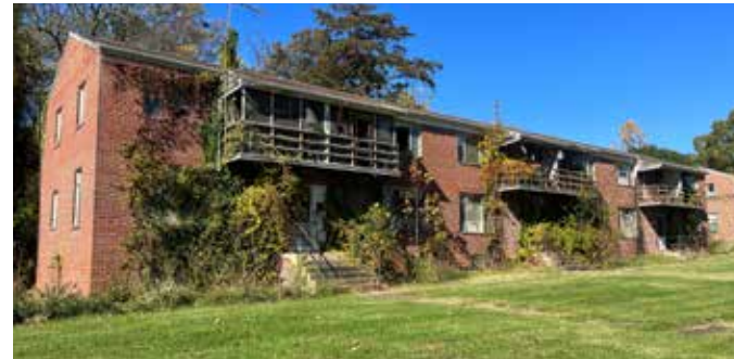
Employee Apartment B | Credit: EHT Traceries
