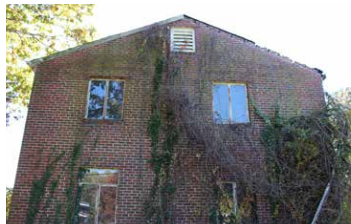
Employee Apartments A - View of Side Elevation - November 2023 - source: Design Collective
