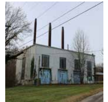
Boiler Plant | Credit: EHT
