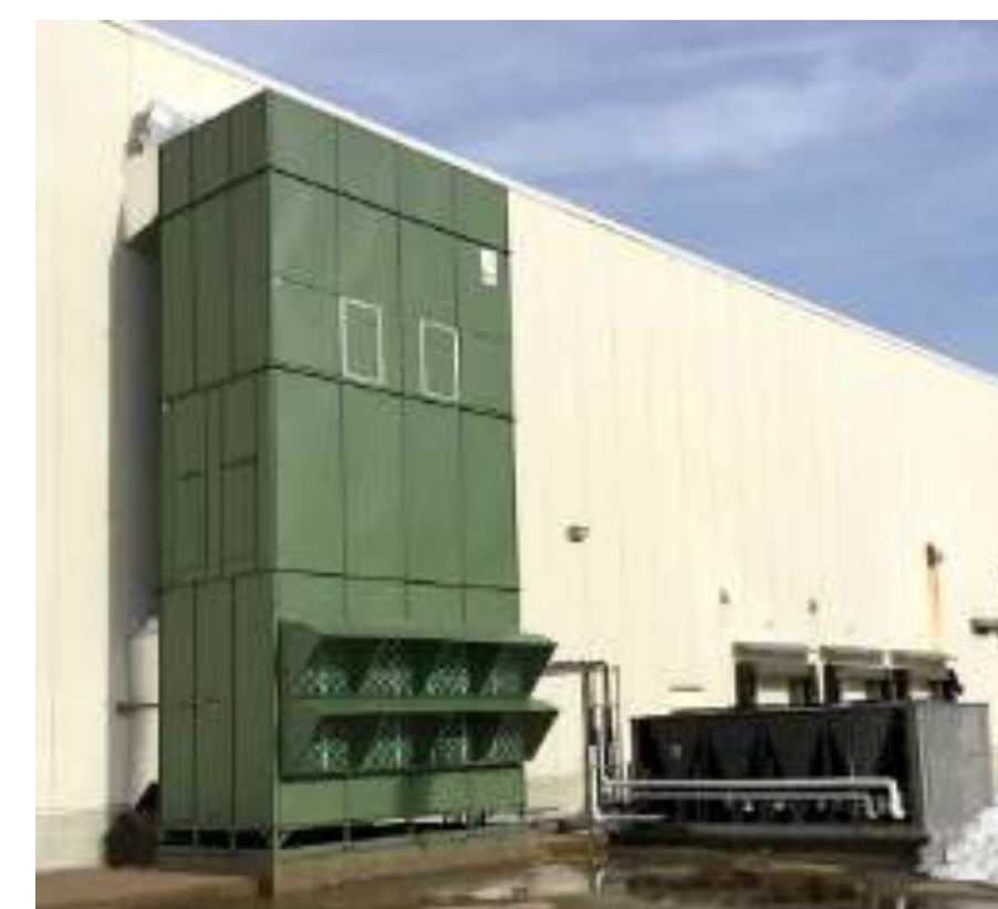
PHOTO OF EXAMPLE AIR ROTATION UNIT (ARU)
