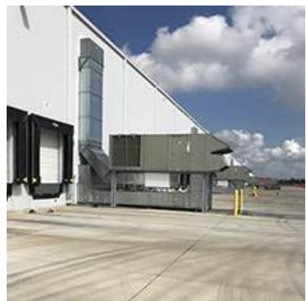
PHOTO OF EXAMPLE GRADE-MOUNTED ROOFTOP UNITS (RTU)
