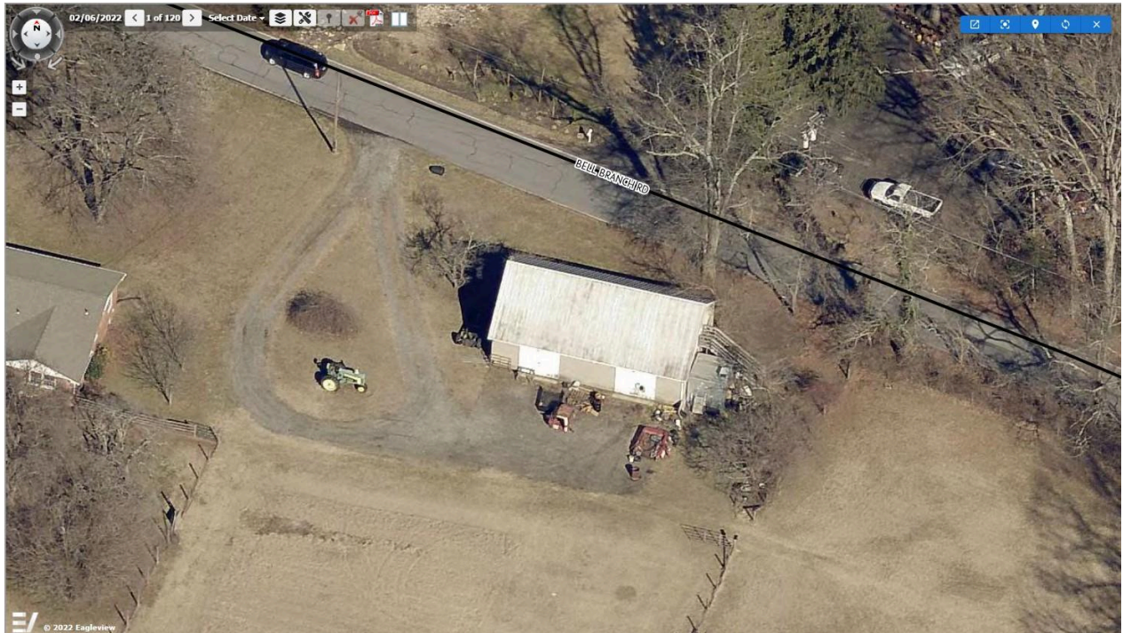
02/06/2022 OBLIQUE AERIAL (facing north) - stairs to upper level of barn, prior to deck
